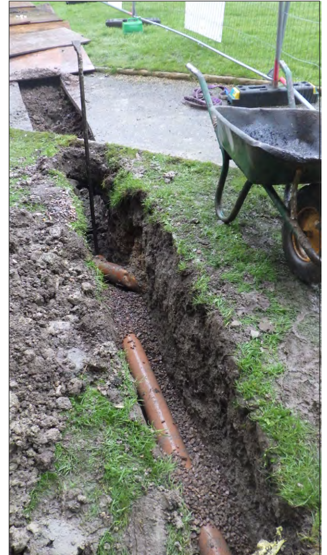
Trench B viewed from the east
