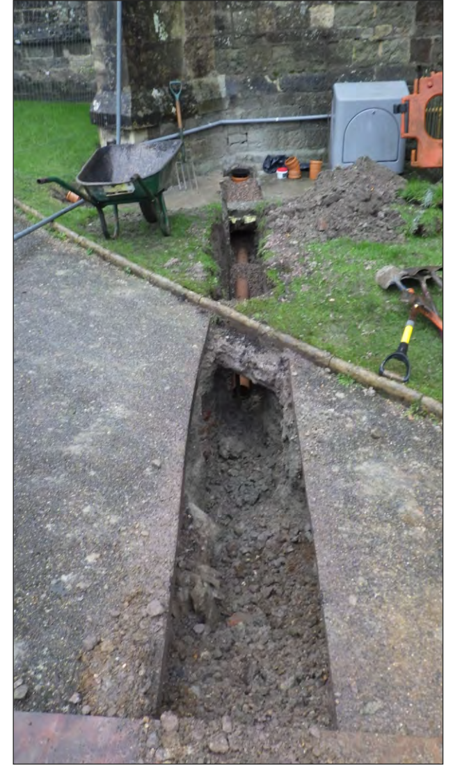
Trench B viewed from the west
