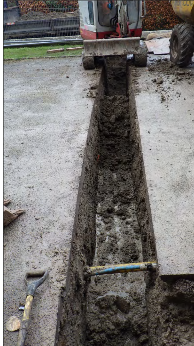
Trench A viewed from the east
