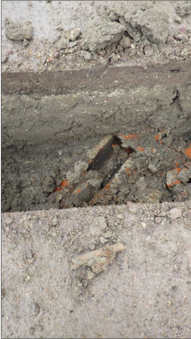
Trench A brick culvert
