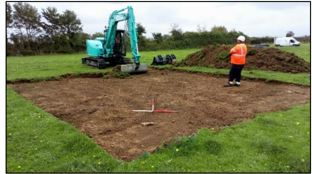
Plate 3. L/R5 area strip in progress Scale: 2x1m
