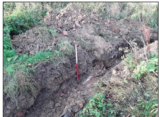
Plate 5. Open-cut trench Scale: 1m
