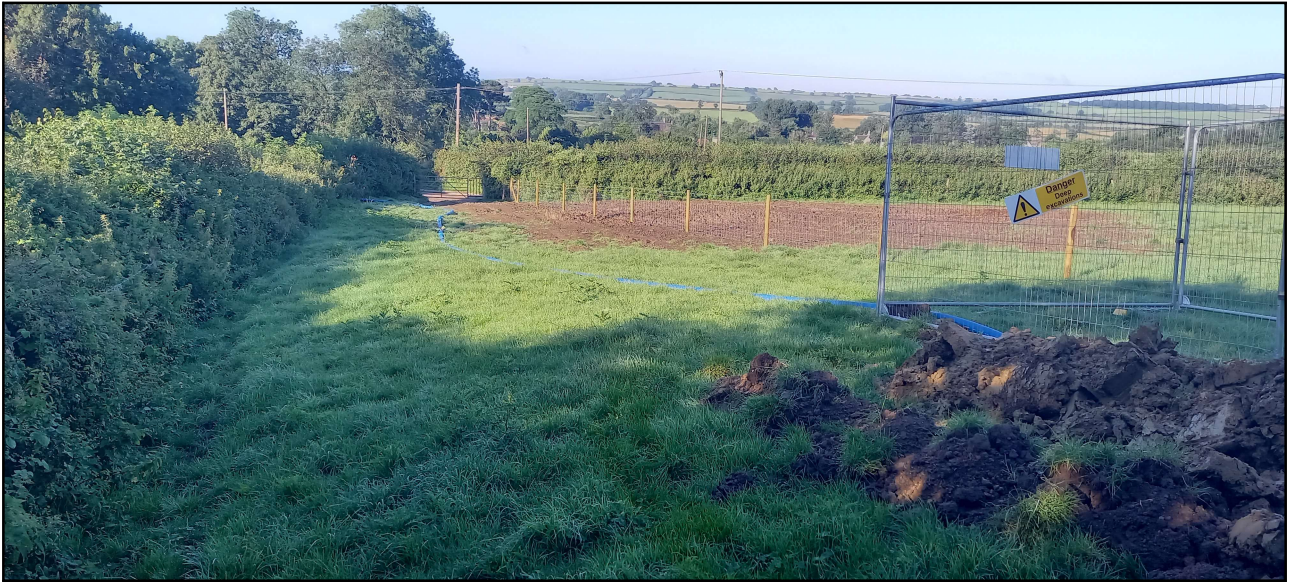
Plate 1: General view of groundworks
