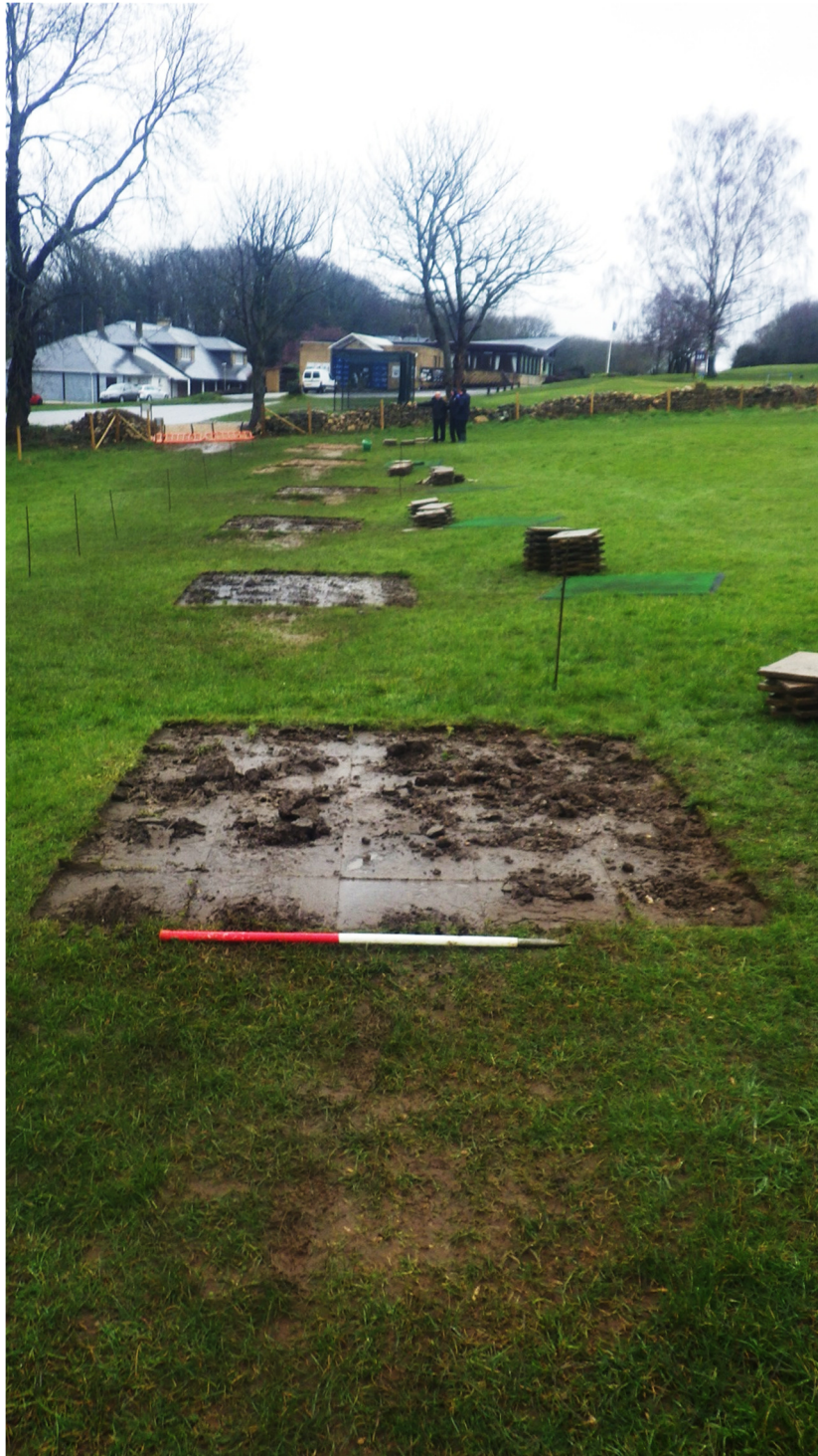
Plate 1: General shot of teeing area following removal of slabs, facing north
