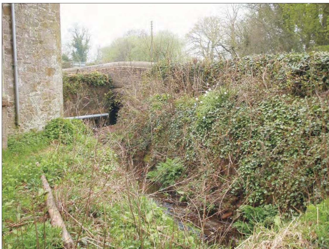
Plate 6: Newland Mill leat, B14. View to northwest.
