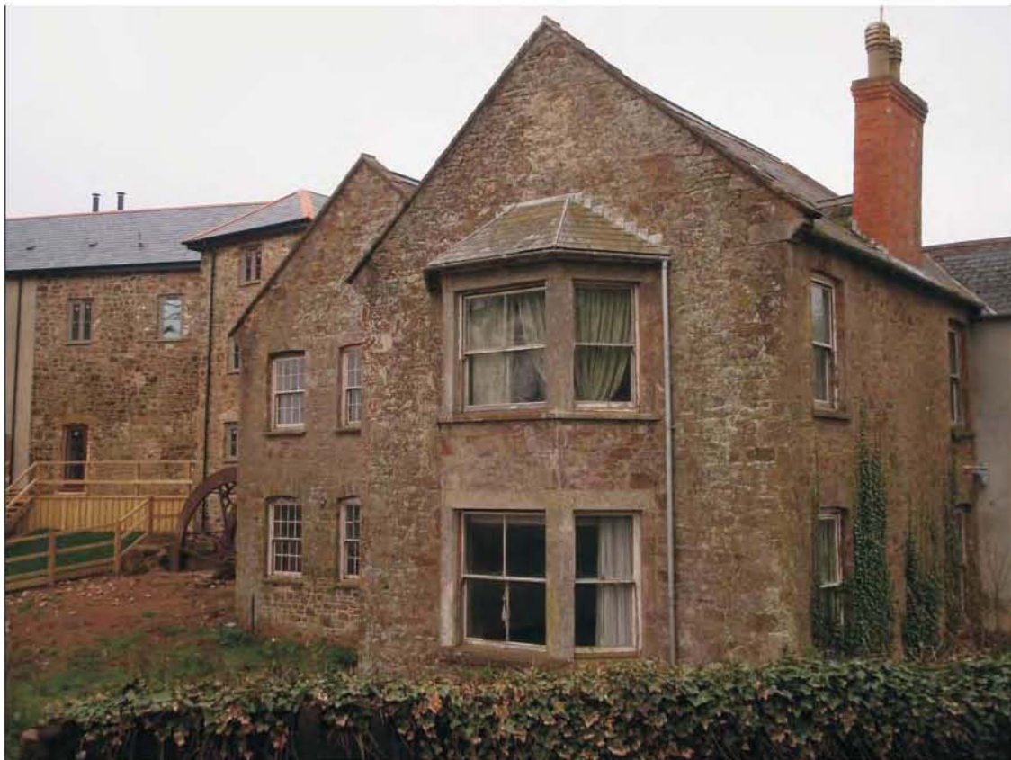
Plate 3: Newland Mill house, B9, with Newland Mill, B8, in background. View to south
