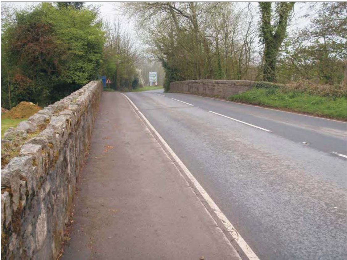
Plate 2: Newland Bridge, B10. View to west
