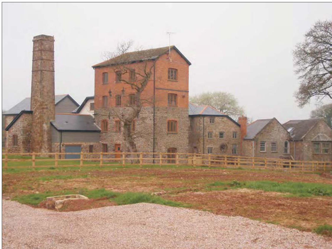
Plate 5: Newland Mill, B8. View to southwest
