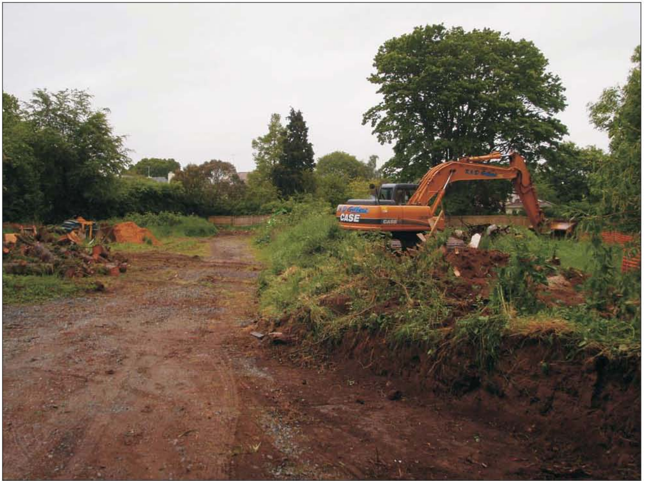
Plate 1: General view of site, looking to north
