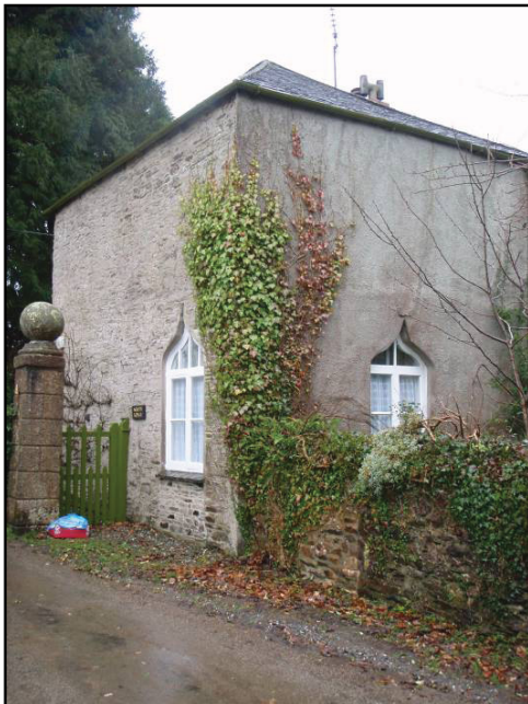
Plate 2: South Lodge and gate pier (Site B6) to Moditonham Park
