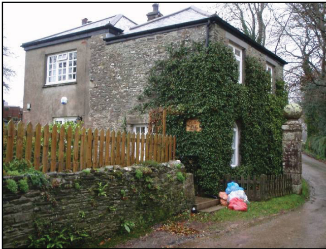
Plate 1: North Lodge and gate pier (Site B6) to Moditonham Park
