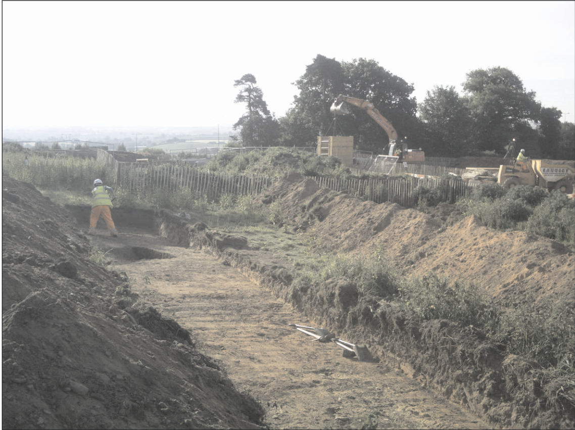
Plate 1: General view of site from Trench 2, looking to southeast
