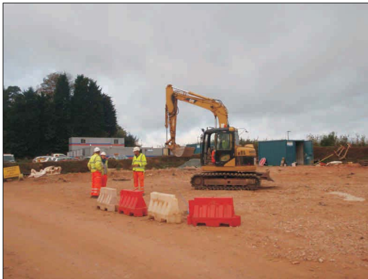
Plate 1: General view of site, looking to northwest
