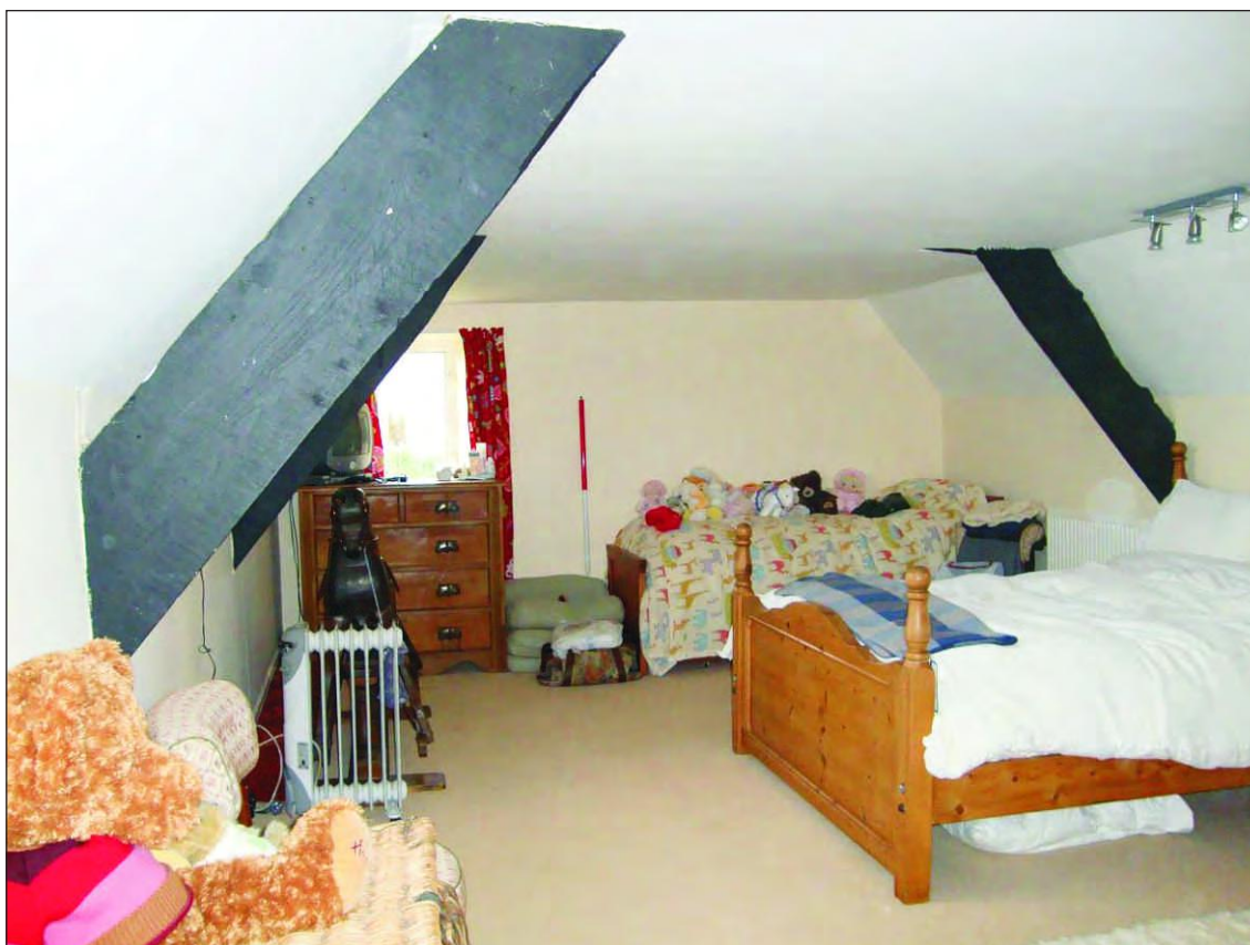
Plate 10: View within the attics, looking west, showing the substantial blades of the principal rafters (Scale 1m)
