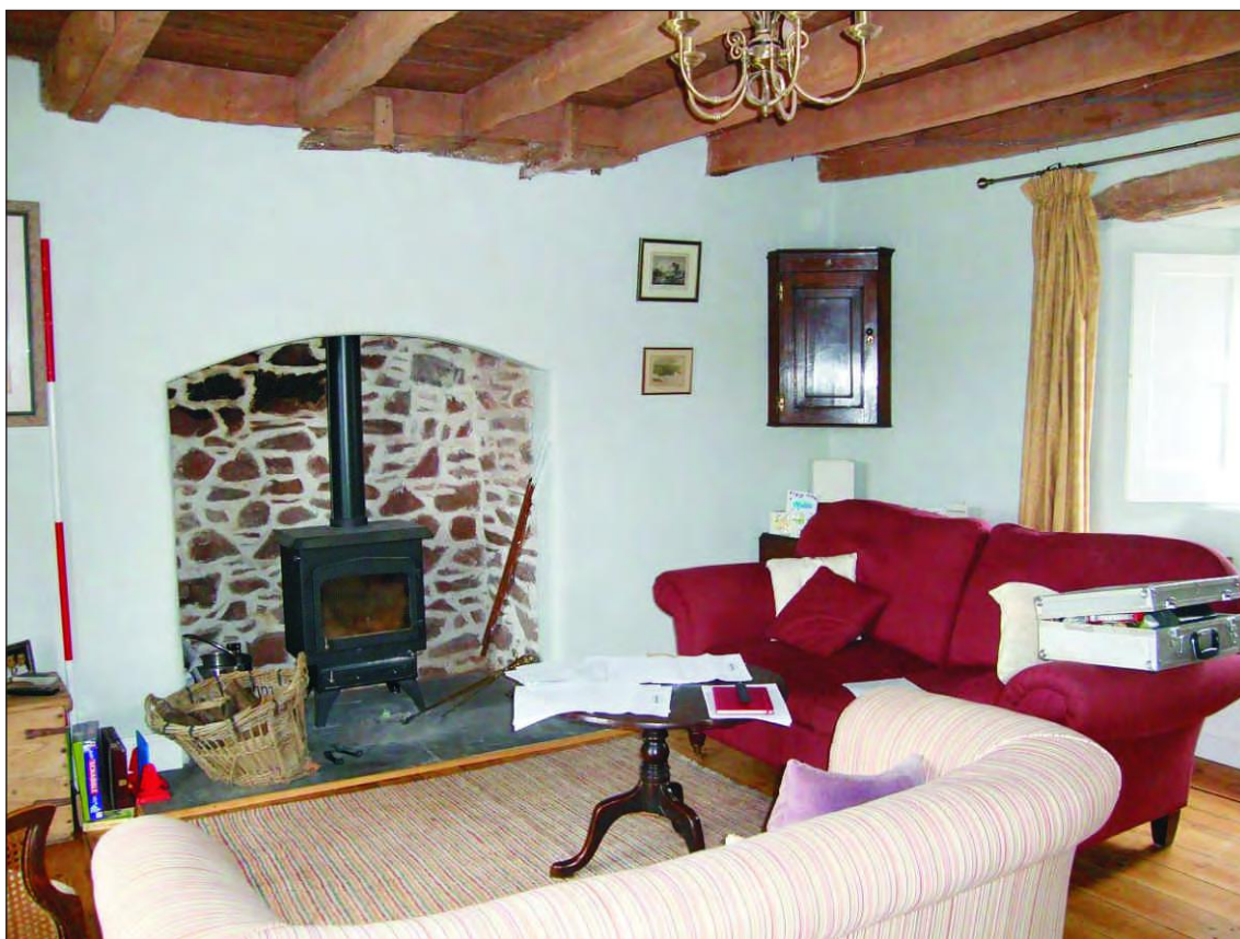
Plate 6: View within the drawing room showing the modern fireplace, exposed ceiling joists and the shutters to the northern window (far right) (Scale 2m)
