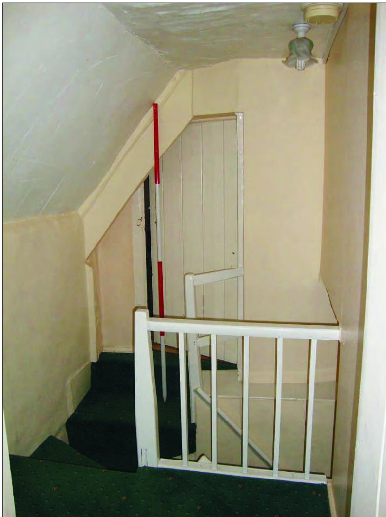
Plate 9: View of the summit of the staircase on the second floor showing the complex arrangement at the stair head, suggestive of alterations (Scale 2m)
