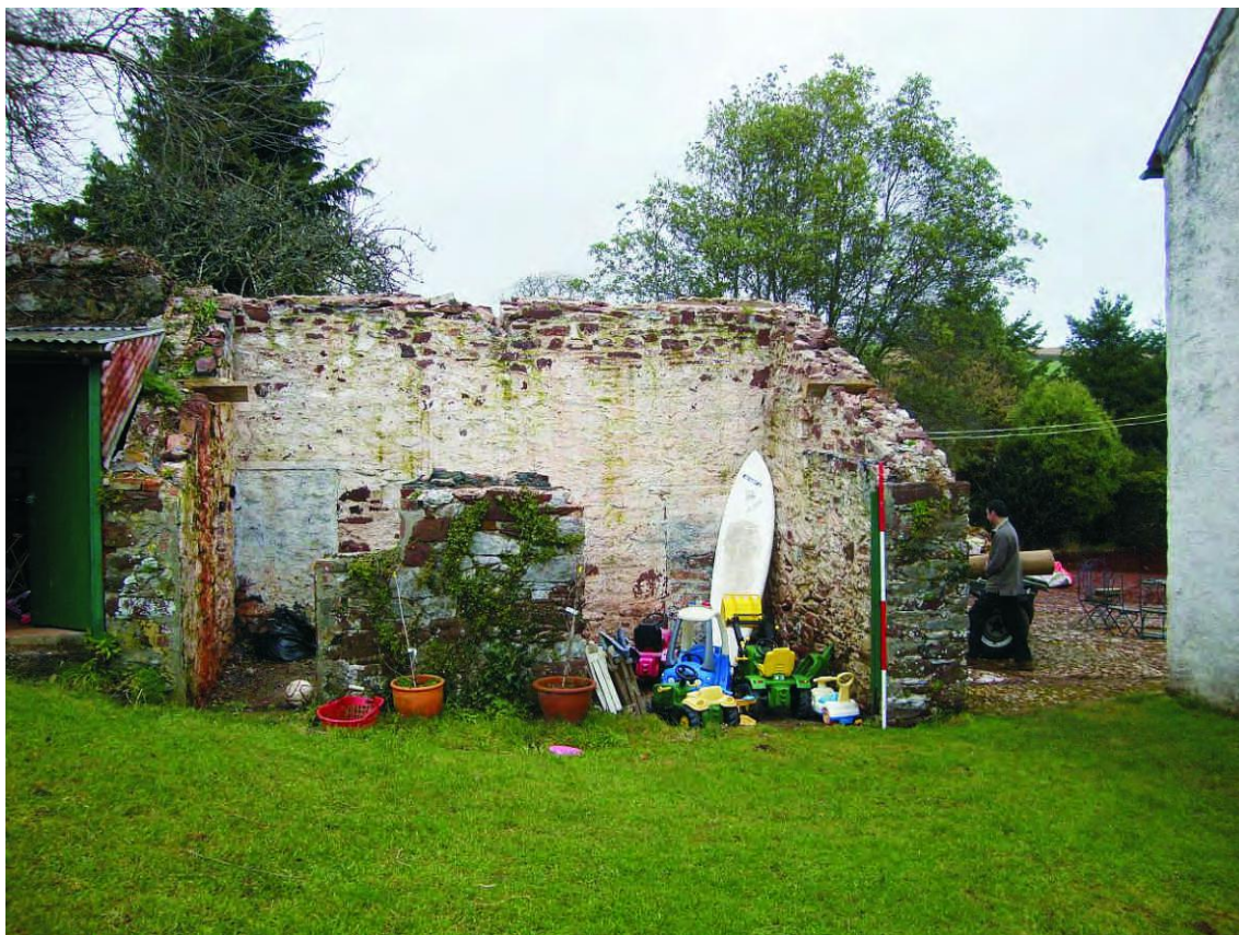
Plate 15: The remains of the pigsty to the west of the house, showing the blocked openings in the rear wall of the building, which formerly opened into a larger structure, now demolished (Scale 2m)
