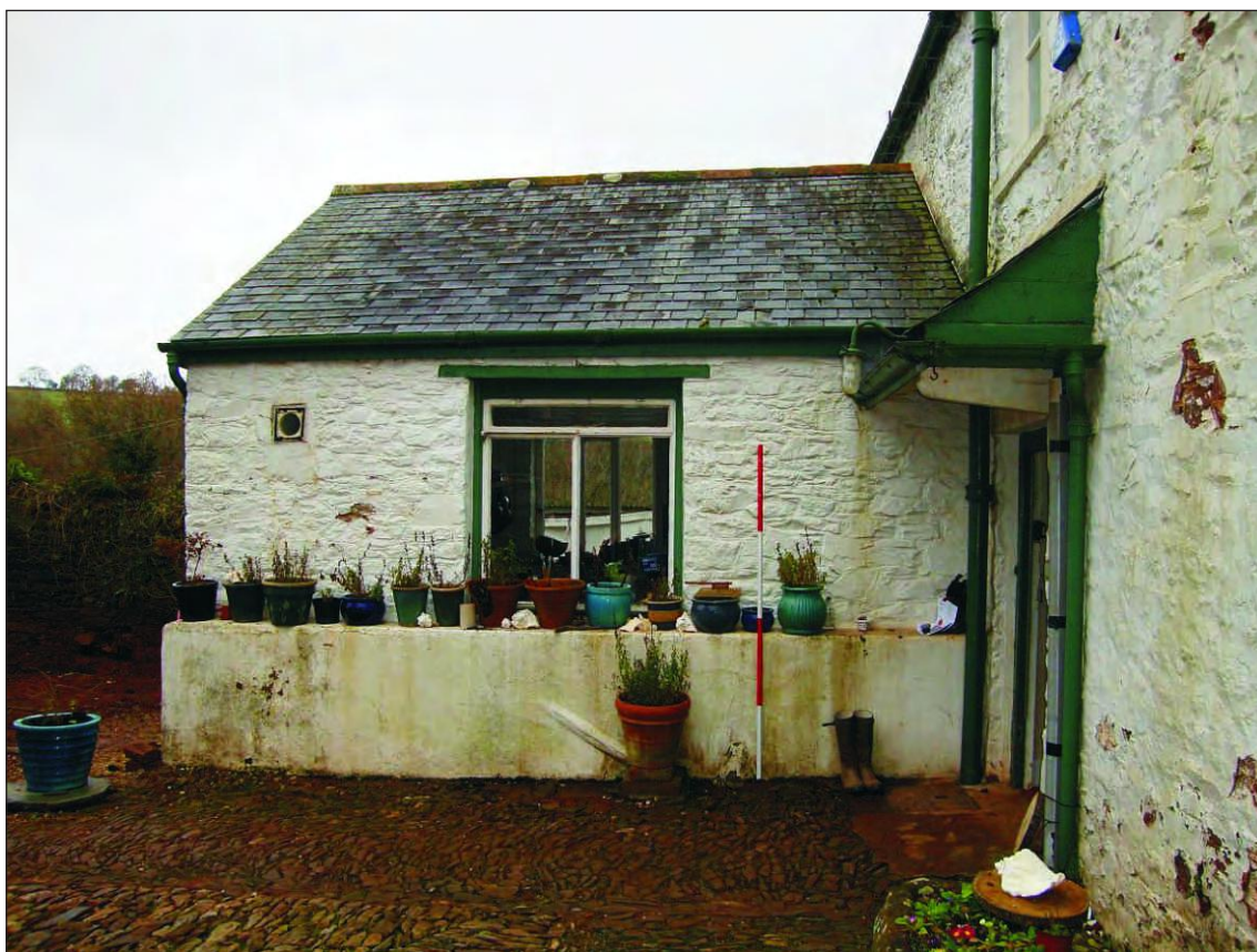
Plate 4: View of the western elevation of the north wing, showing the projecting plinth at the base of the wall and the metal-framed 'Crittall' window in the upper section (Scale 2m)
