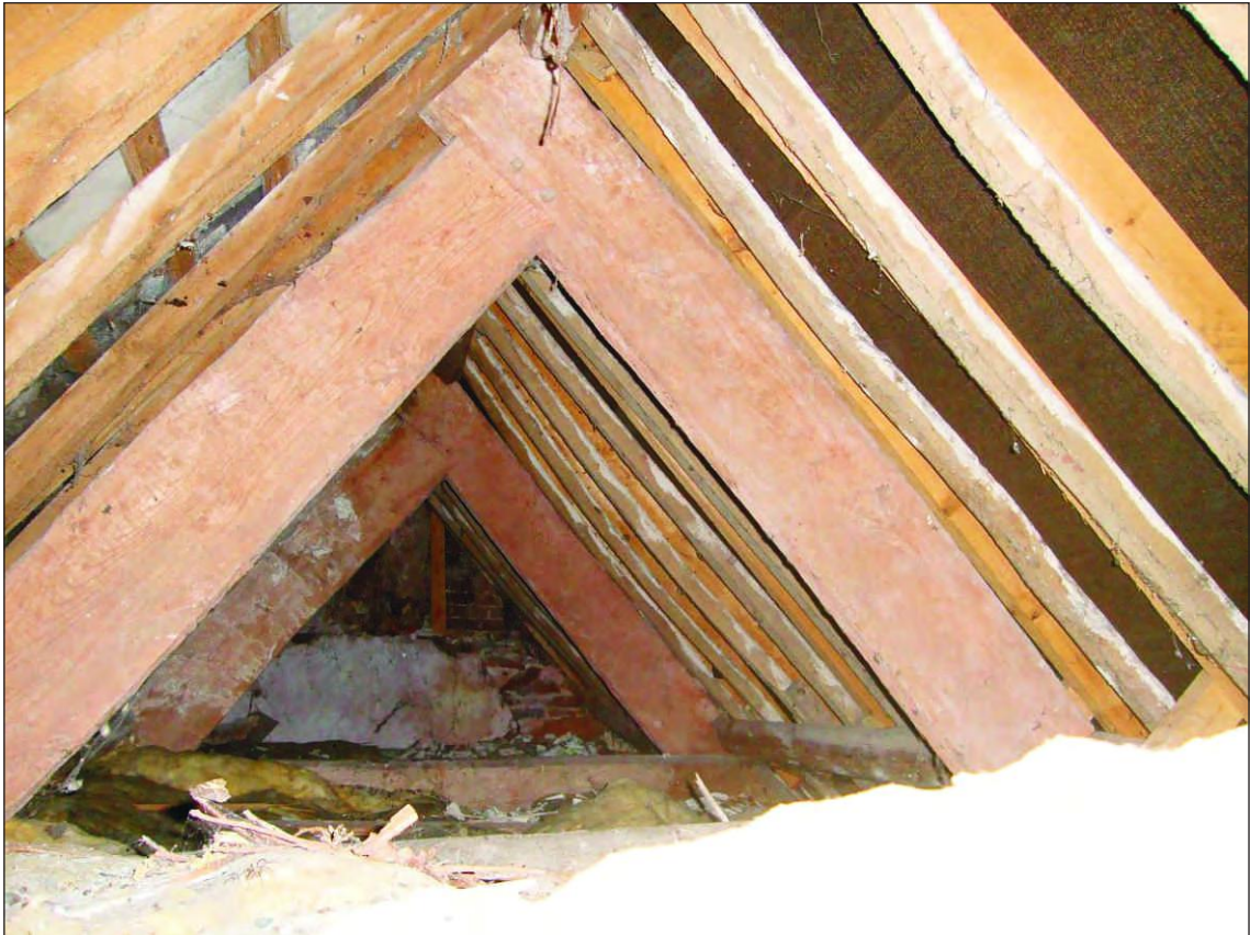
Plate 11: View within the roof space, looking west, showing the substantial roof timbers and evidence of plastering on the interior of the west wall
