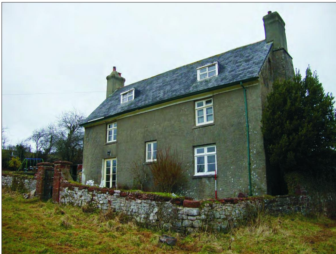
Plate 1: View of the south façade of the house, looking north west, showing the coved cornice beneath the eaves and the late 19th or early 20th century fenestration (Scale 2m)
