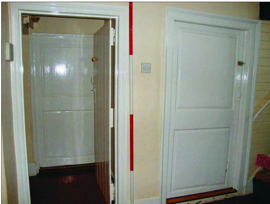
Plate 5: Details of the 18th century panelled doors in the hallway, showing the door to the dining room and the later lobby to the left (Scale 2m)
