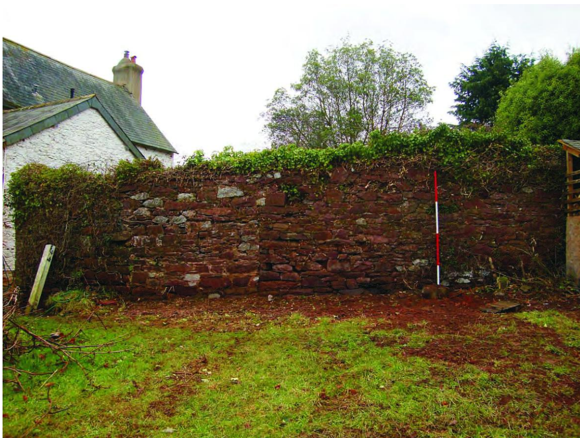
Plate 16: Part of the wall, lying to the north of the house, possibly connected with the demolished northern range of farm buildings. A blocked gateway lies just left of centre (Scale 2m)
