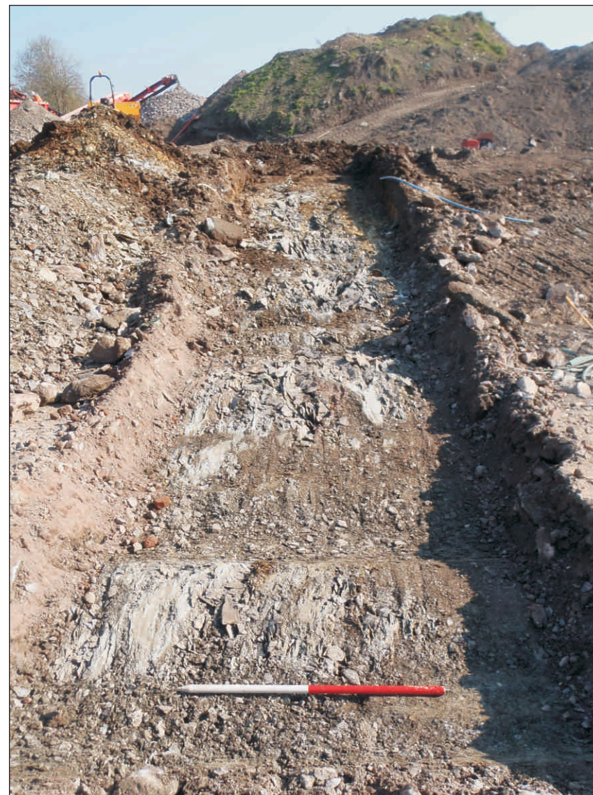
Plate 2: Trench 3 showing terrace for Woodhey Road in the foreground, viewed from the west-southwest. Scale 1m
