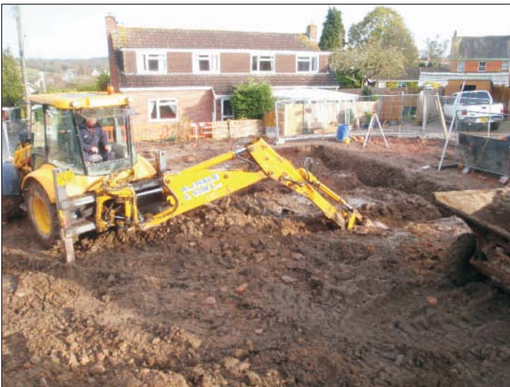
Plate 3: Excavation of foundation trenches during watching brief, looking northeast
