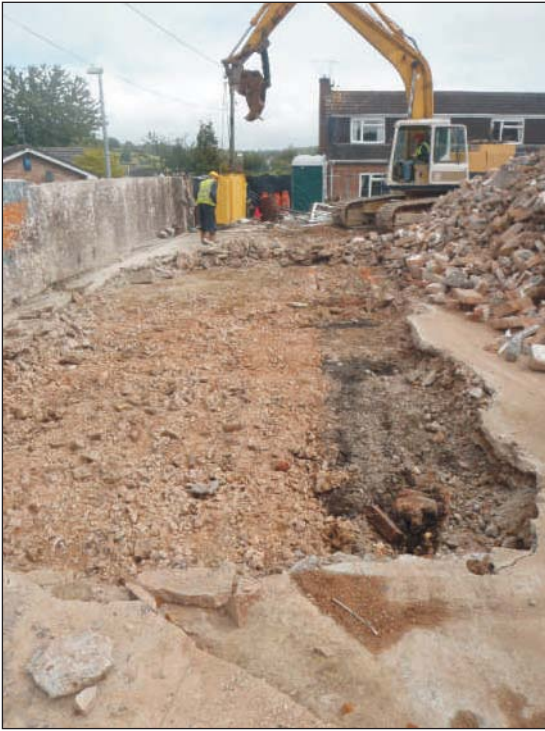
Plate 1: Removal of concrete slab, view to northeast
