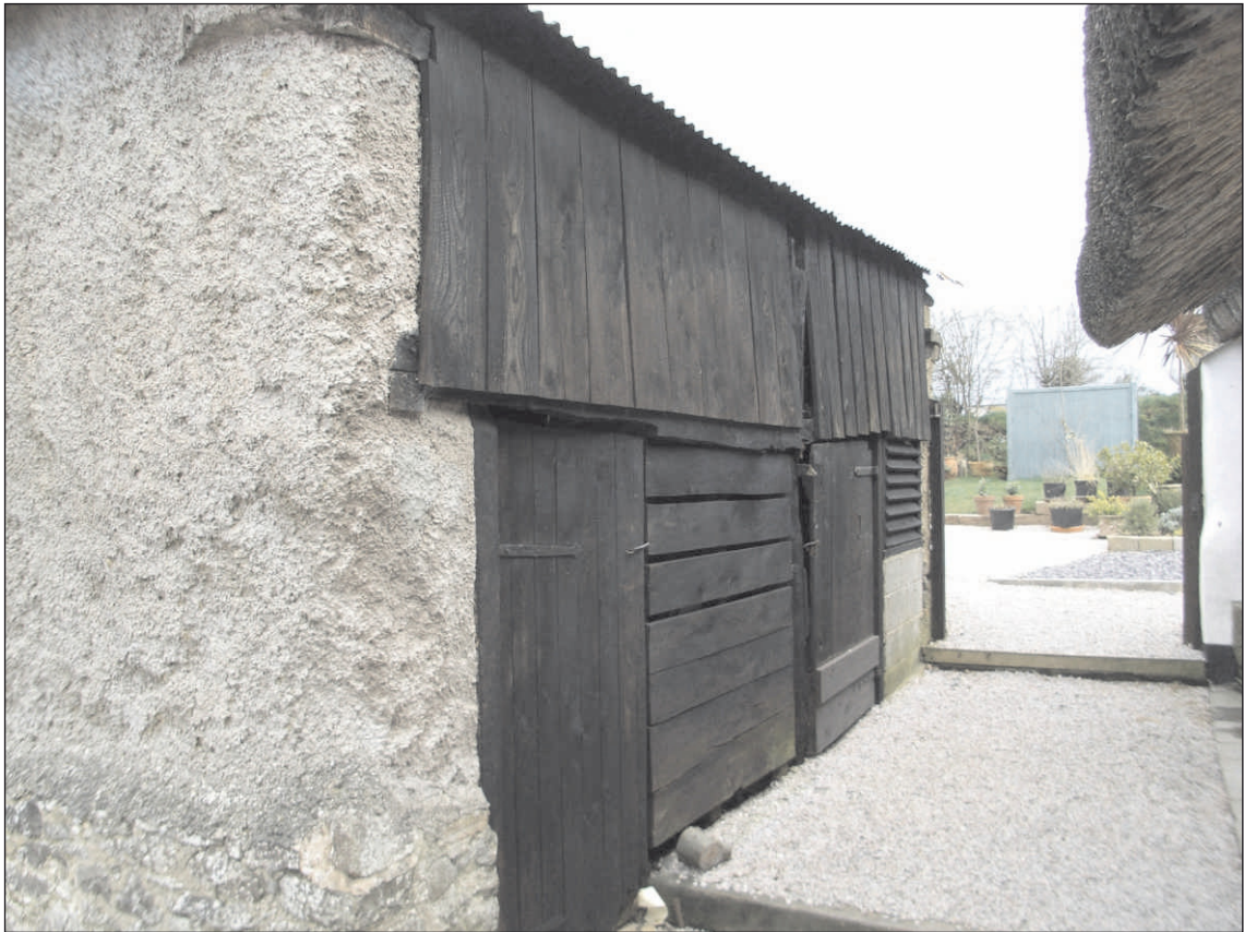
Plate 3: The south elevation of the barn, looking to northeast.
