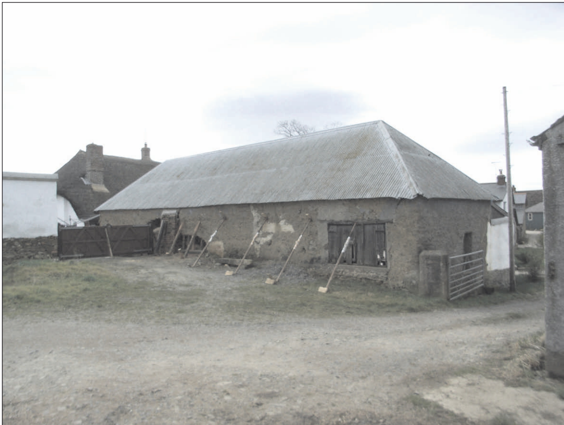
Plate 2: The east elevation of the barn, looking southwest.
