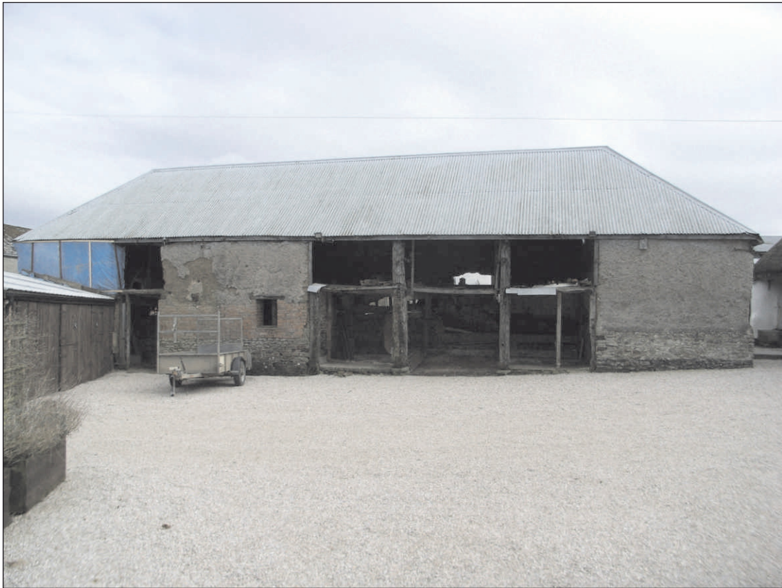
Plate 1: The west elevation of the barn, looking east.
