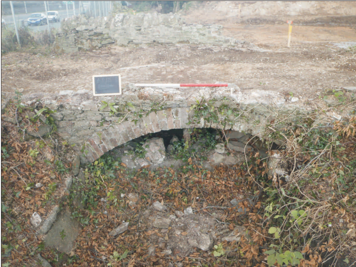
Plate 3: South elevation of bridge. View from the south. Scale 1m
