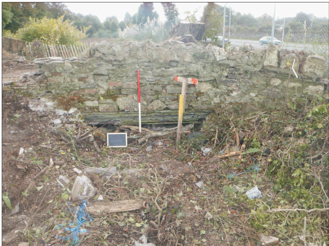
Plate 2: North elevation of bridge (secondary phase). View from north. Scale 1m
