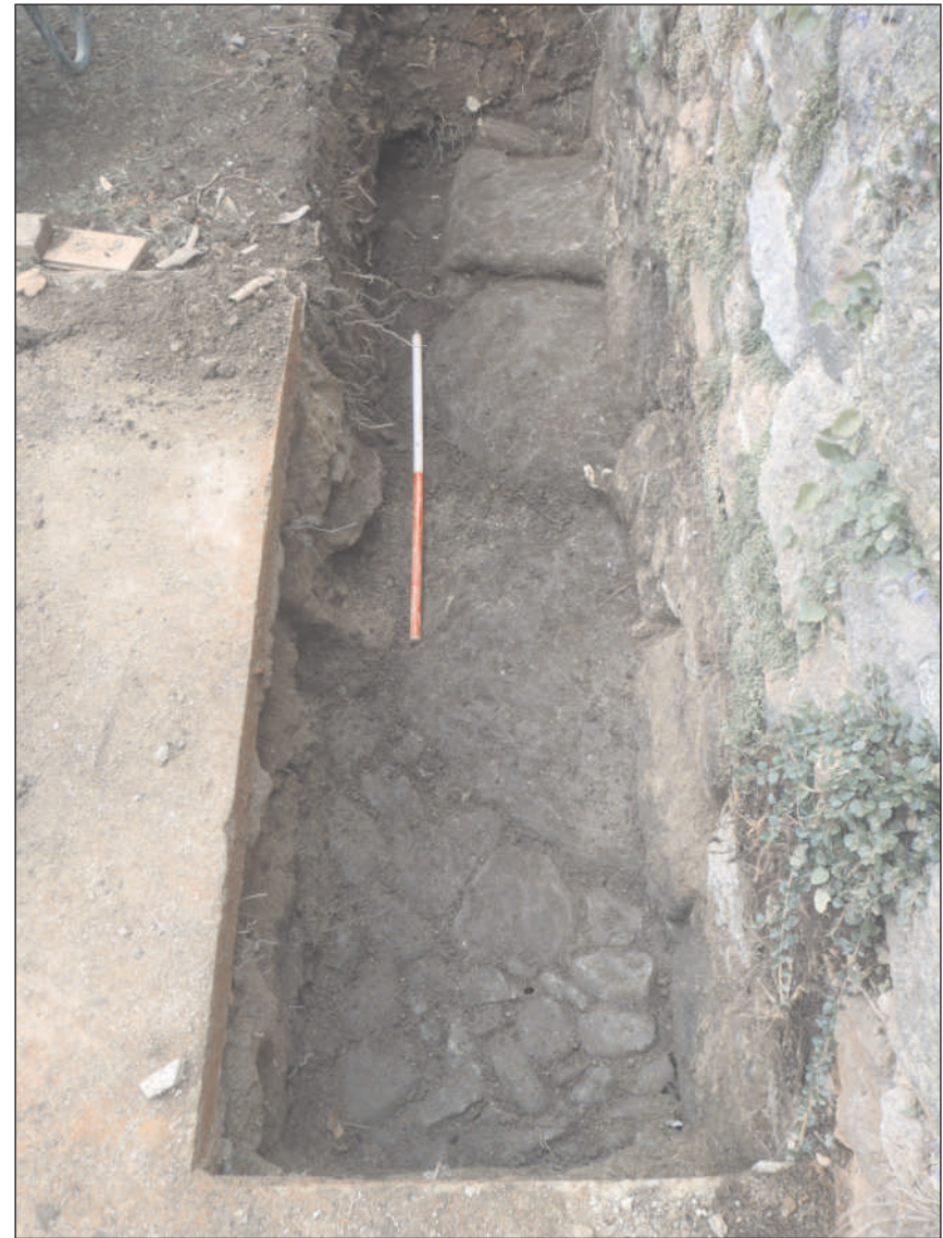
Plate 4: The foundation trench showing the footings of the shippon (107) and later cobbles (103), viewed from the south. (1m scale)
