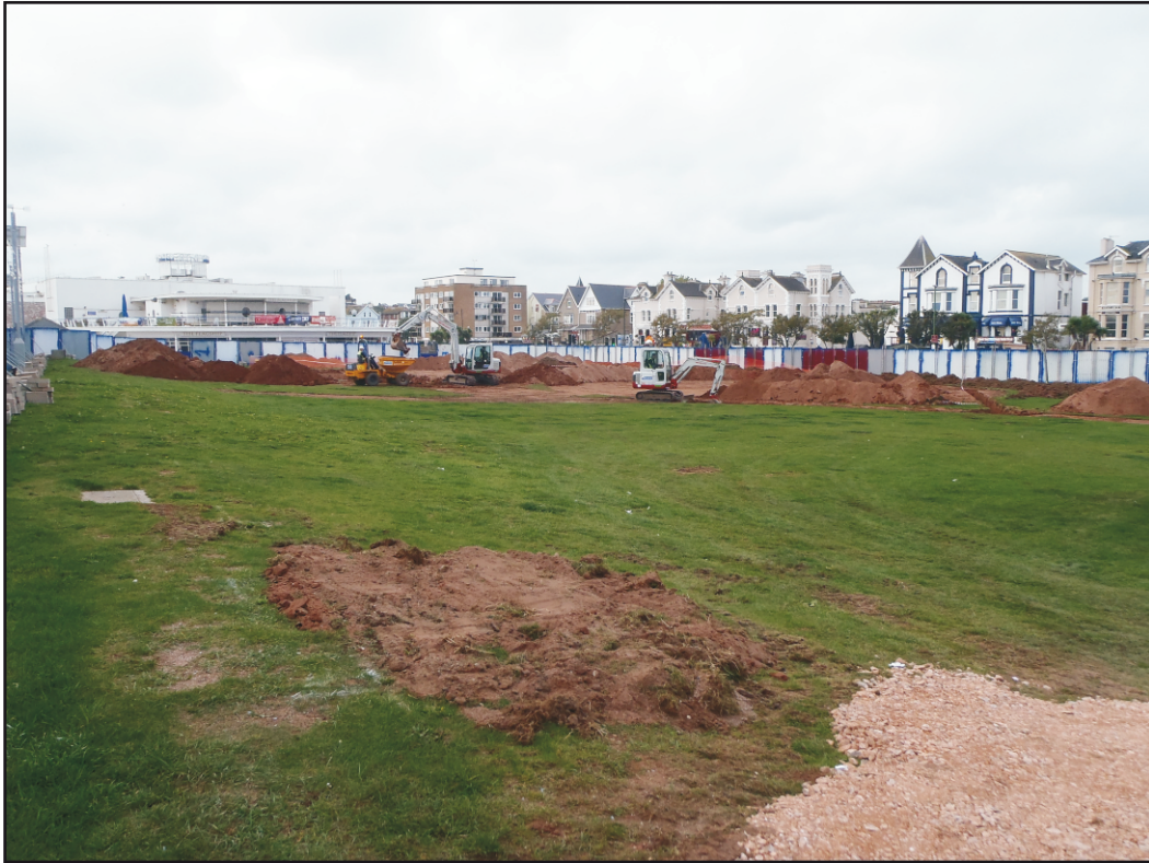
Plate 1: General view of site, viewed from the North
