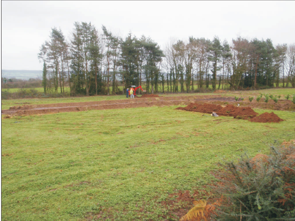
Plate 1: General view of site, looking southeast
