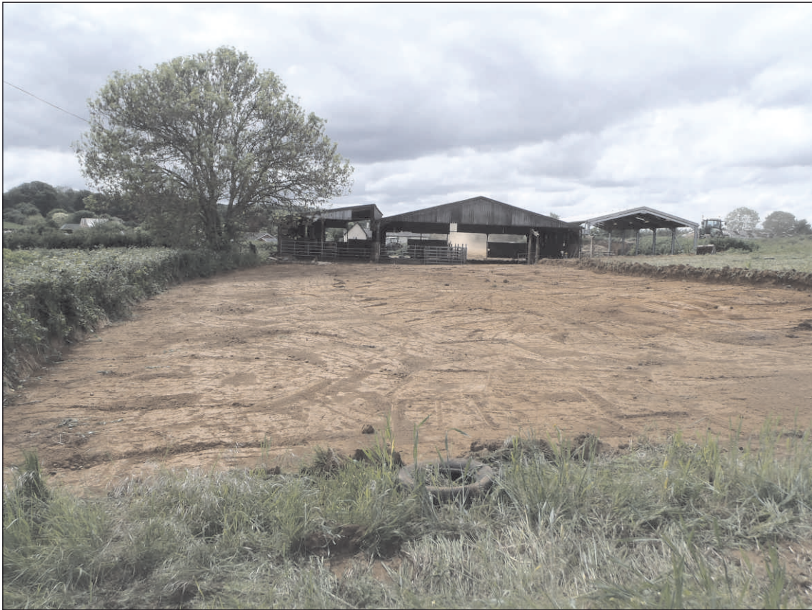
Plate 2: General view of site after topsoil stripping, view to southwest.
