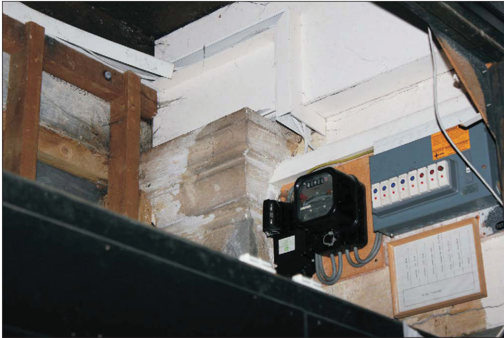
Plate 3: Close-up view of a stone capital in the central front column, viewed from the southwest.
