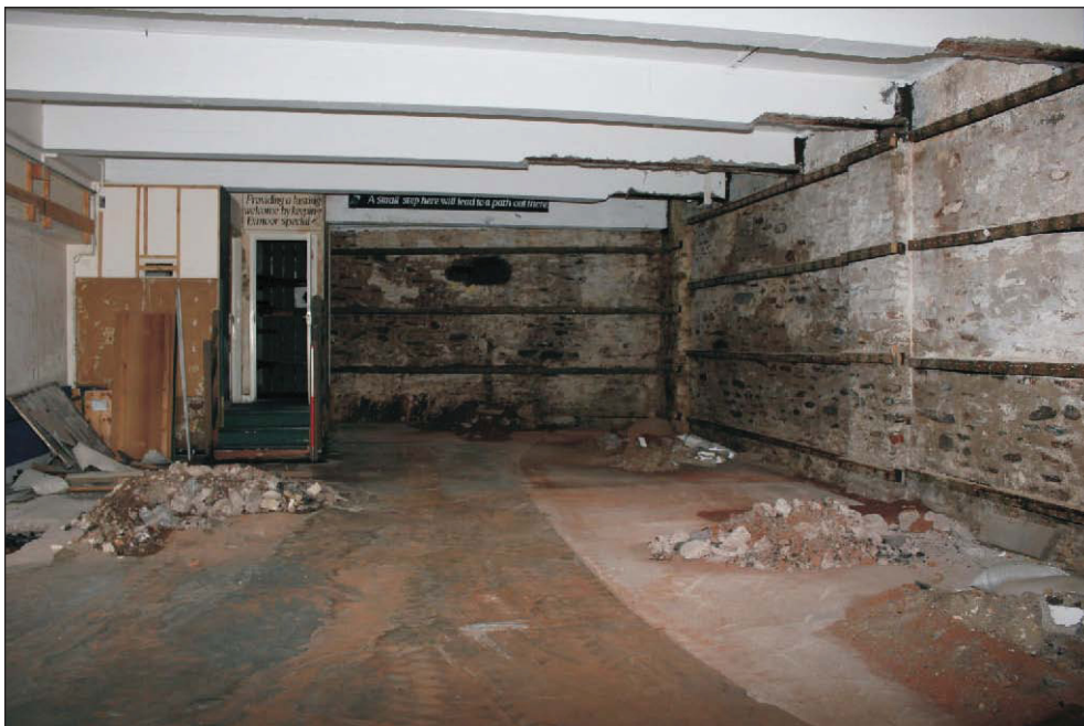
Plate 2: The ground-floor west room, viewed from the north. 1m scale.
