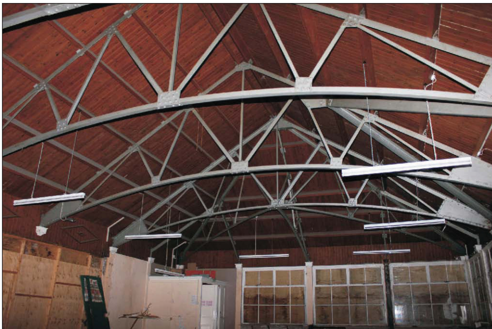
Plate 10: The roof trusses, viewed from the east.
