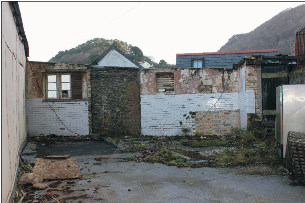
Plate 8: The former men's toilets and stage, viewed from the west. 1m scale.
