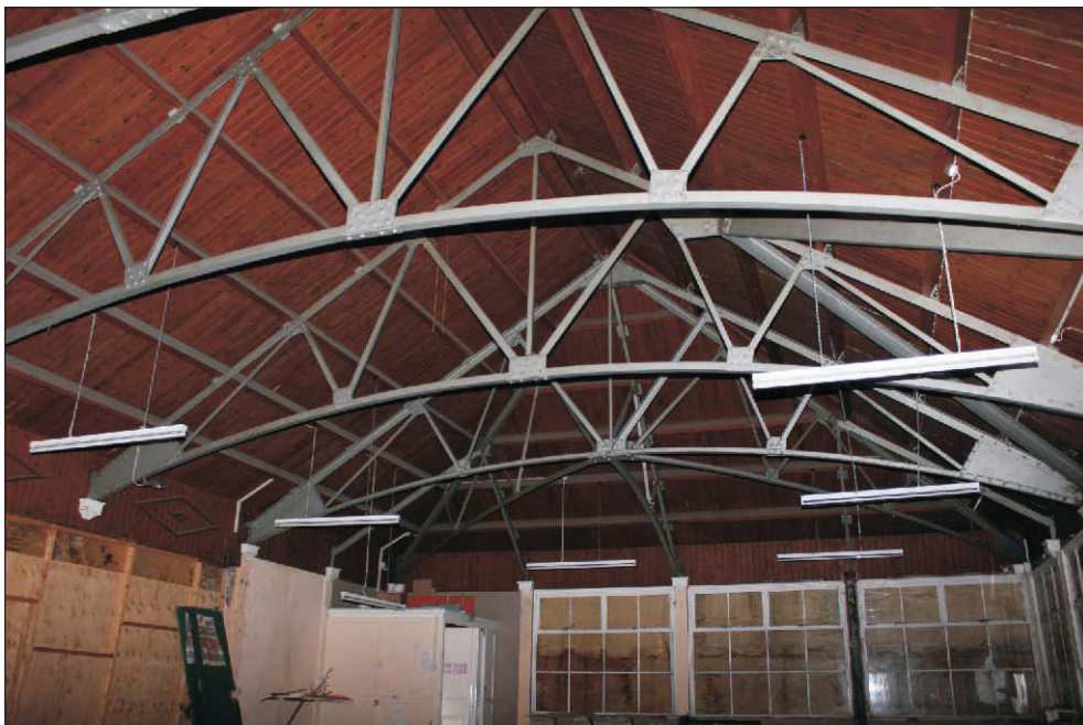
Plate 10: The roof trusses, viewed from the east.
