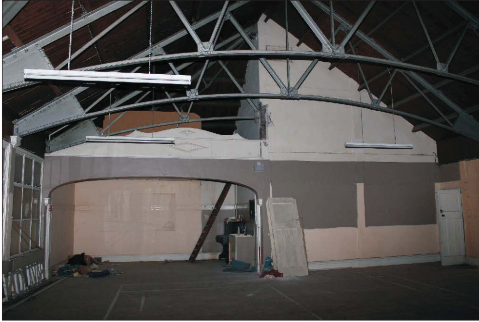
Plate 7: The first floor showing the store area and lighting box at the east end, viewed from the west. 1m scale.
