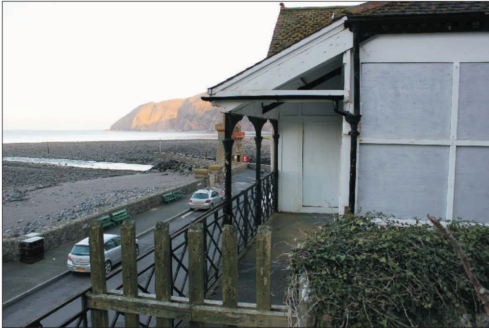
Plate 9: The western balcony, viewed from the west.
