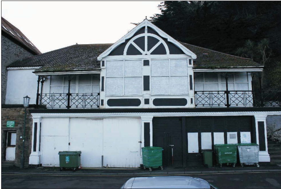
Plate 1: The front elevation, viewed from the north. 1m scale.
