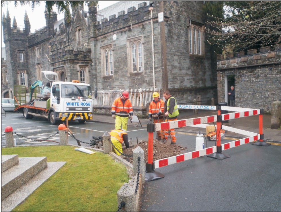
Plate 1: Trench 1 under excavation. View to northeast
