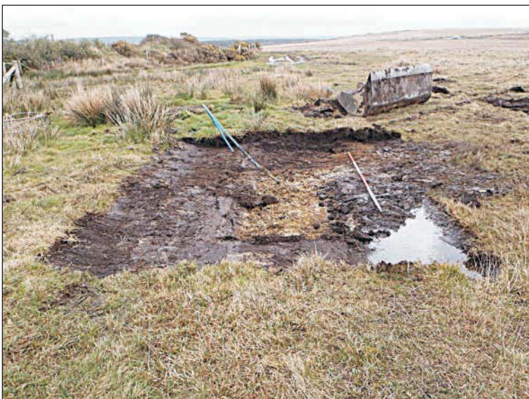
Plate 3: The excavation for the resited trough. View to the northeast (2m scale).
