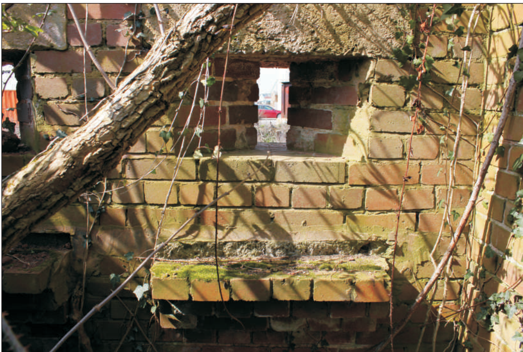
Plate 4: Pen 145, defended wall, interior view showing rifle step. View to northwest.
