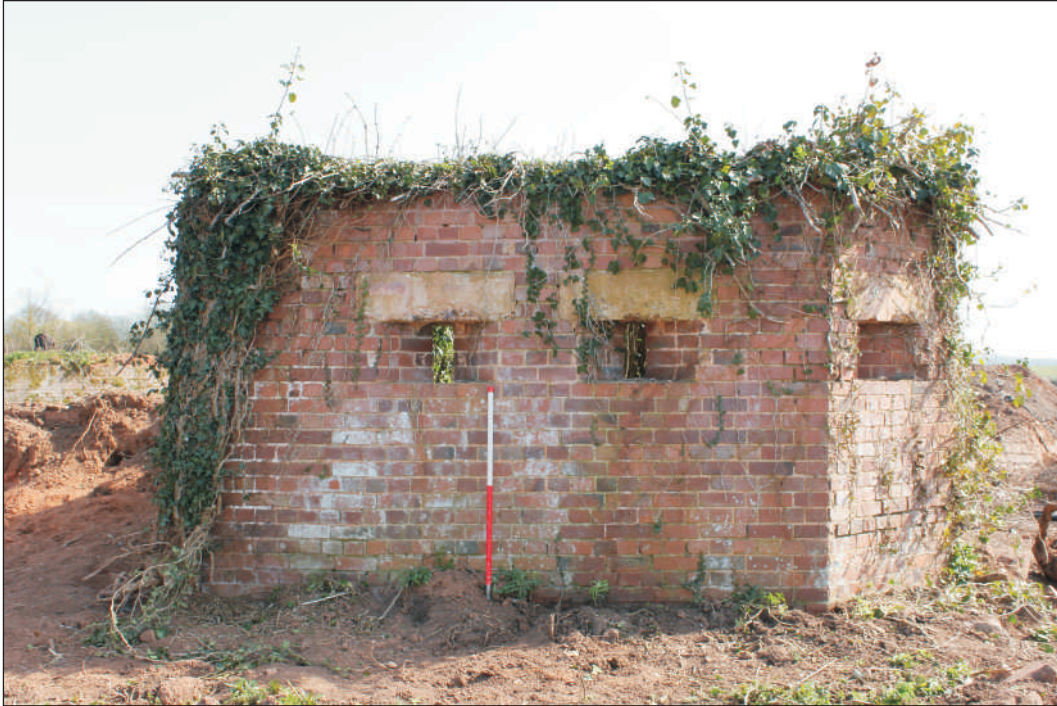
Plate 3: Pen 145, defended wall, west elevations. View to east. 1m scale.
