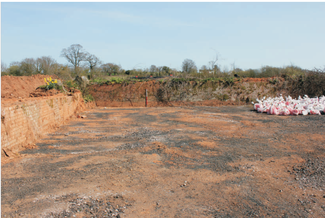
Plate 2: Pen 145, general view of west bay showing difference in heights of retaining walls. View to east. 1m scale.
