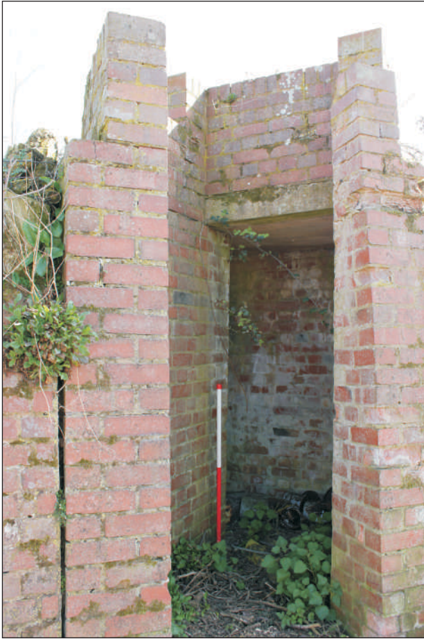
Plate 5: Pen 145, west entrance to air raid shelter. View to southeast. 1m scale.
