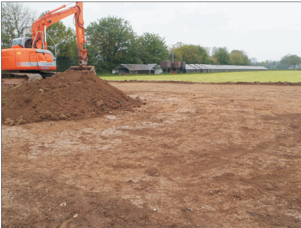
Plate 2: General view of groundworks. Looking northwest
