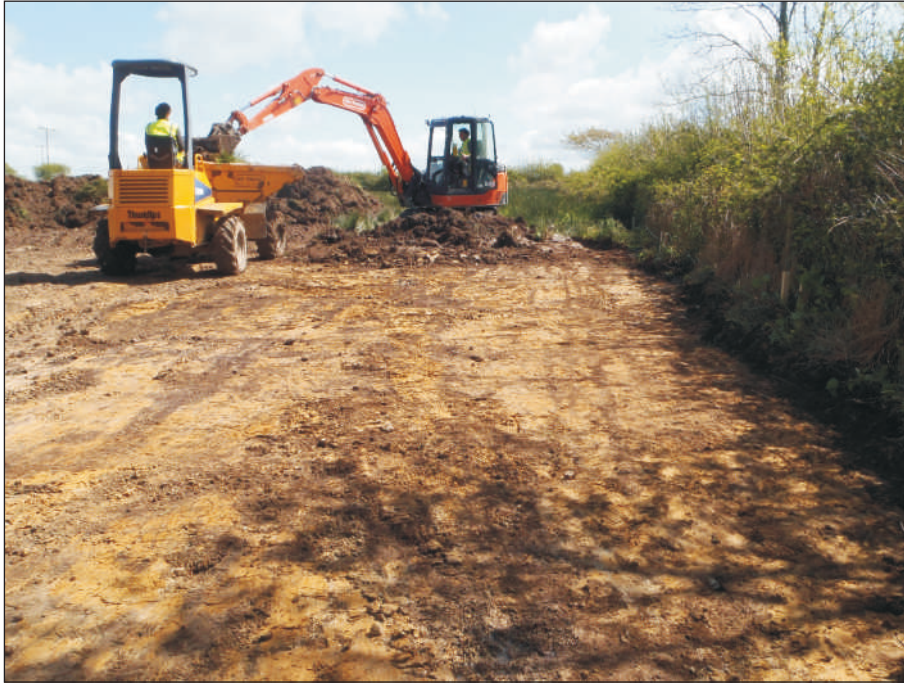
Plate 1: General view of site, showing plough scarring parallel to hedgebank. View to southwest
