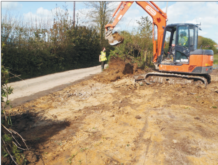
Plate 2: Removal of roadside hedgebank. View to northeast
