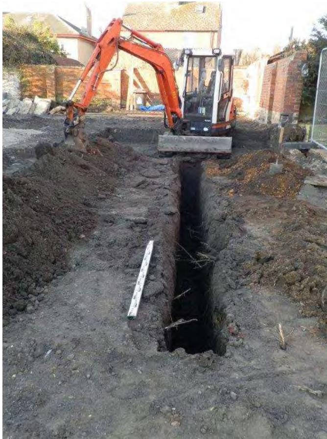
Plate 1: View of trench from the east
