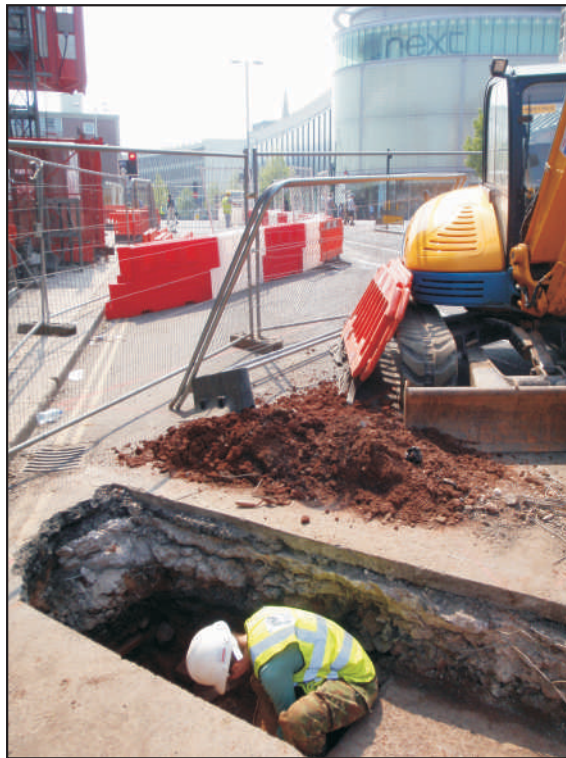
Plate 1: Working shot of site, viewed from the WNW.
