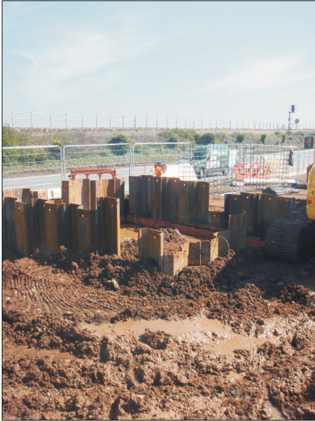
Plate 1: General view of launch pit looking southeast
