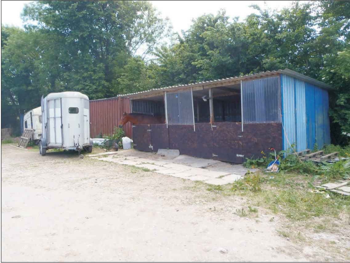
Plate 1: Southwest end of the application area (view from northeast)
