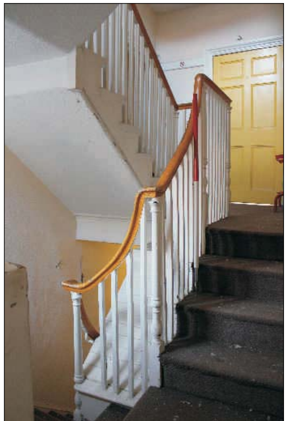
Plate 7: The staircase looking from the southeast towards the first floor. Scale 1m.
