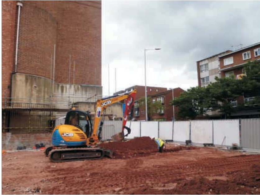
Plate 5: General view of site looking from the west.
