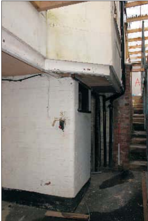
Plate 12: Coal cellar and courtyard viewed from the southeast. Scale 1m.
