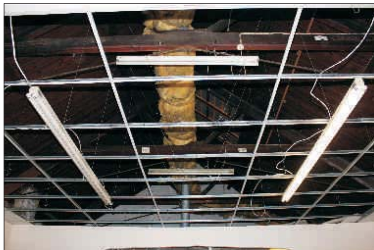
Plate 14: Gymnasium, roof structure viewed from the southeast.
