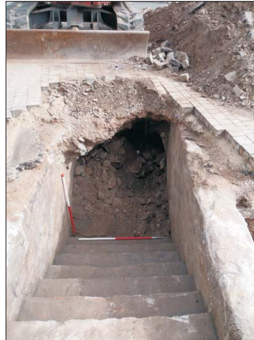
Plate 10: Trench 3. Entrance to air raid shelter. View from the southwest (scale 2 x 1m)
