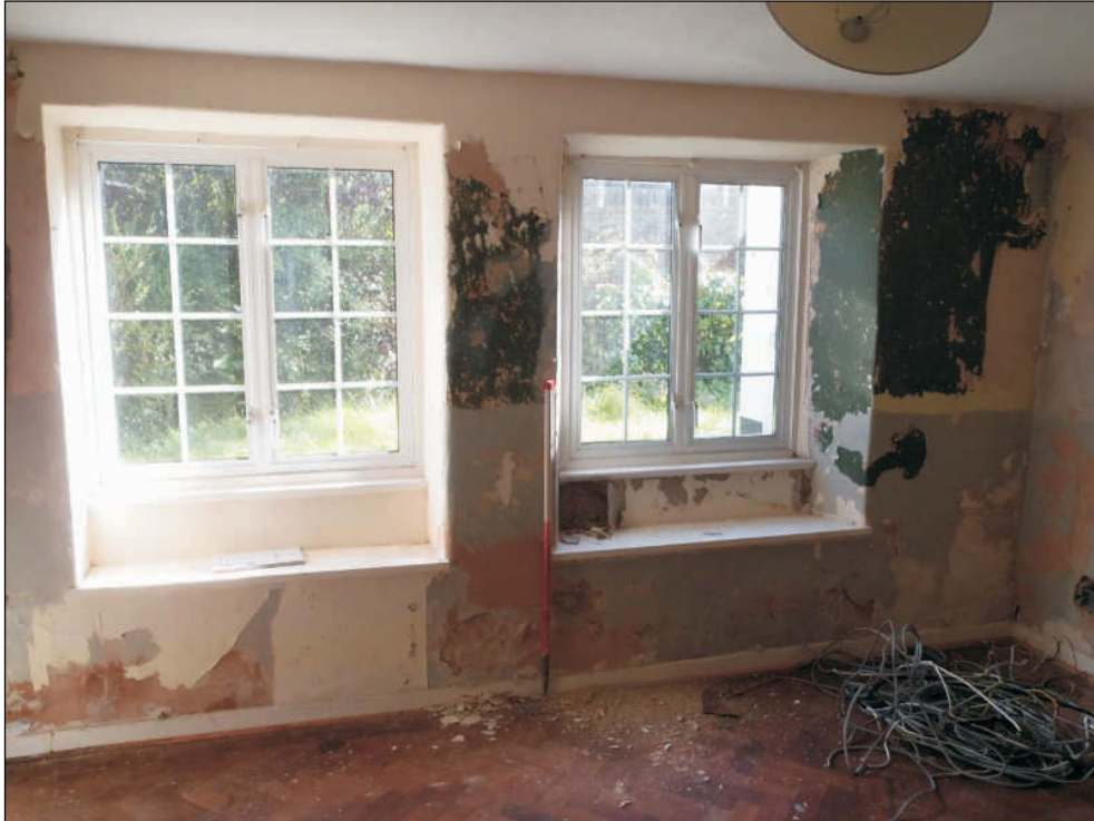
Plate 5: Ground floor primary splayed window opening (right) with former doorway, now a window, to the left, viewed from the southwest. Scale 1m.
