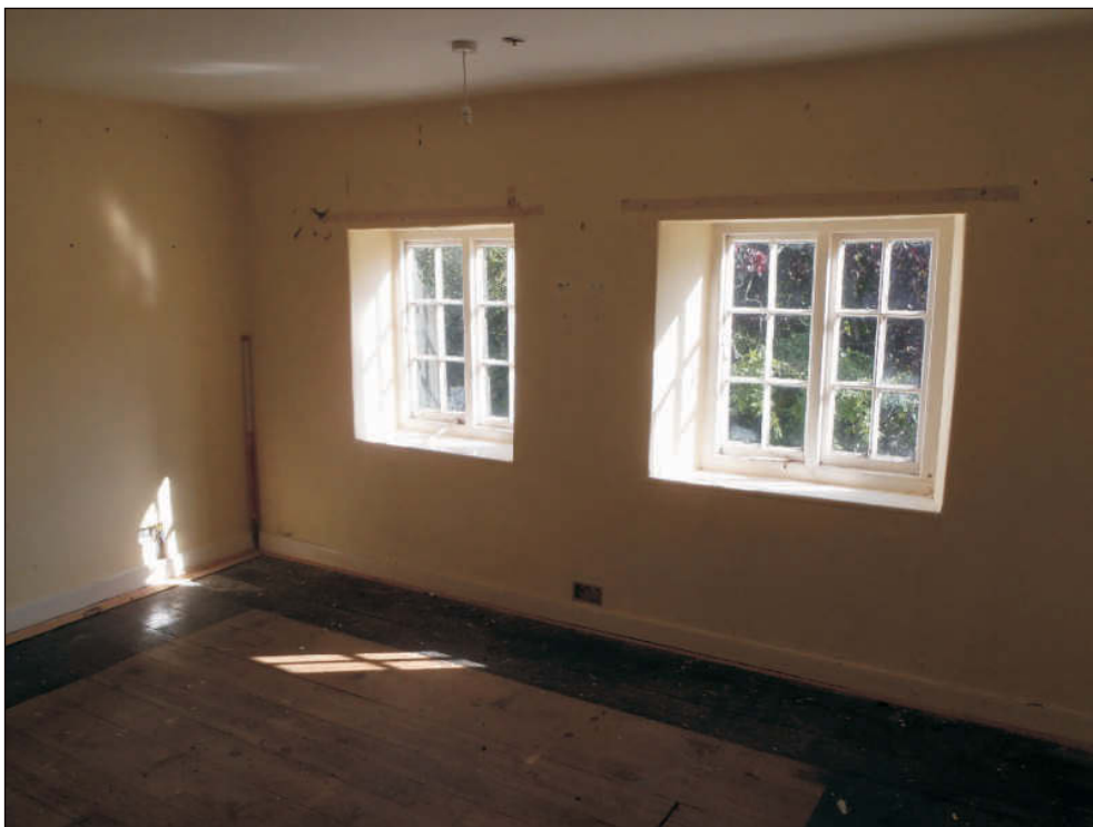
Plate 6: Original first-floor splayed window openings, viewed from the south. Scale 1m.
