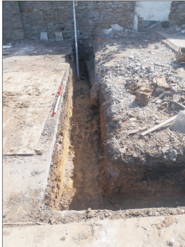
Plate 1: General view of the excavation, viewed from the north. Scale 1m
