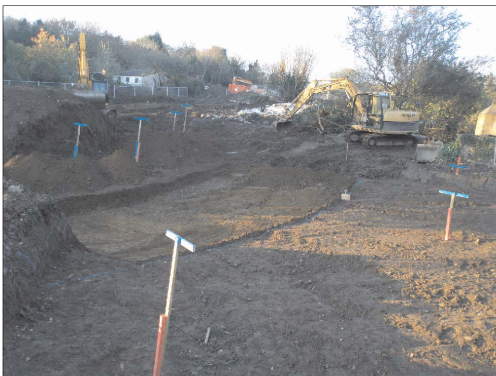
Plate 2: General view of site from the southeast
