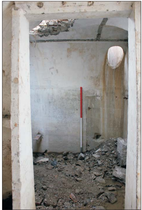
Plate 4: The stove fitting and vent at the south end of the shelter, viewed from the northwest. Scale 1m.
