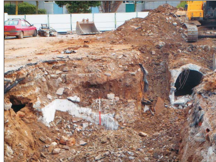
Plate 14: Demolition of air raid shelter. Leat visible to left of scale, view from southwest. Scale 1m
