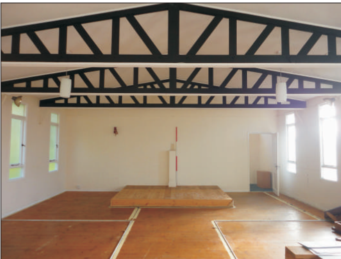
Plate 2 View of the nave of the church, looking east, showing the layout of the former furnishings marked on the floor and the footpace of the altar
