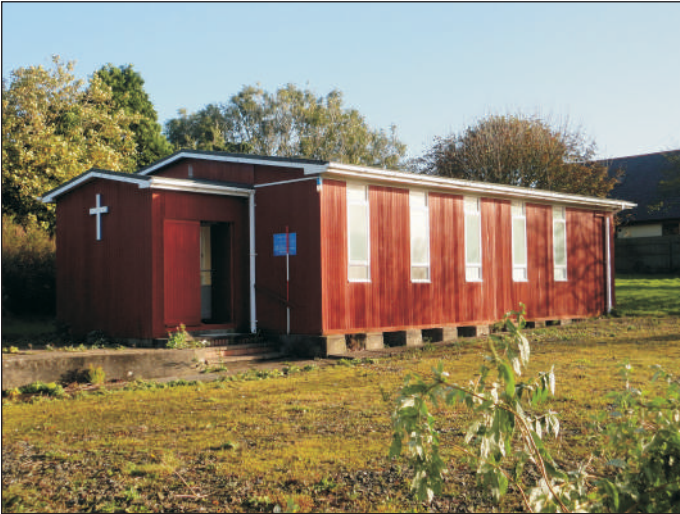
Plate 1 General view of the church from the south west
