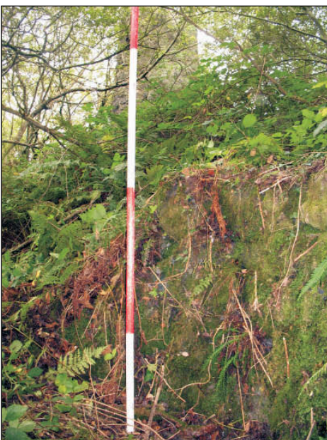
Plate 8: Settling tank No.3, showing the curved northwest corner, with the chimney stack beyond, view from east-northeast. Scale 2m
