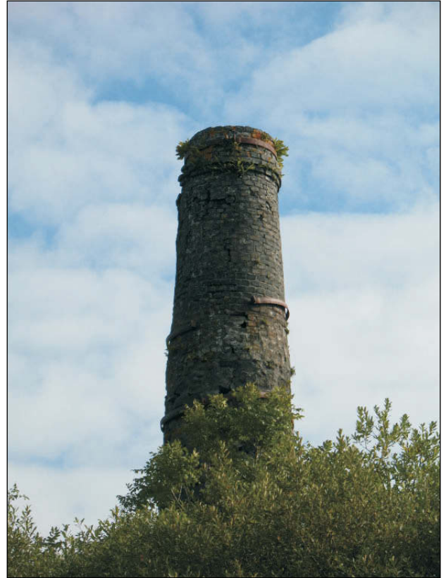
Plate 2: Molinnis chimney top brick courses and iron bands, view from west-southwest
