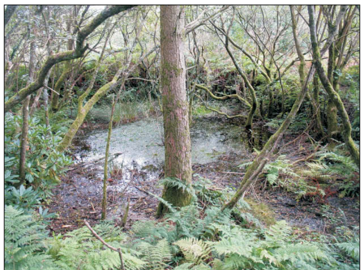
Plate 9: Settling tank No.4, flooded and overgrown, view from NW. This dates from an enlargement of the site sometime in the mid-twentieth century.
