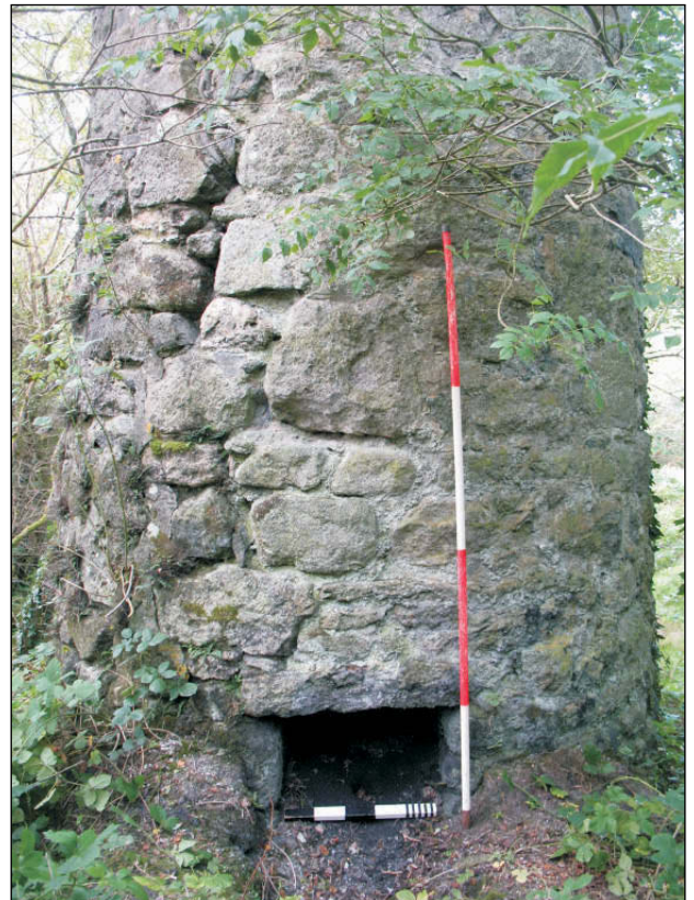
Plate 4: Molinnis chimney base with opening for flue, view from east-northeast. Scales 0.20m and 2m
