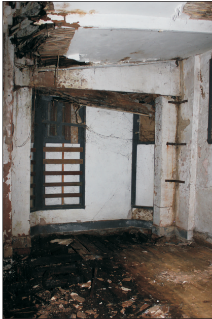
Plate 5: Room 1, bay window in south elevation, viewed from the northeast.
