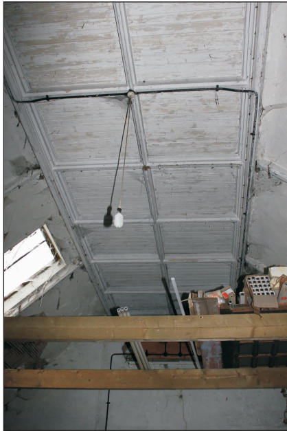
Plate 9: Room 6, the panelled ceiling, viewed from the west.
