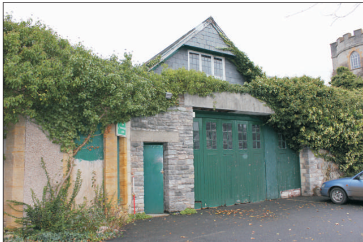
Plate 1: South elevation, viewed from the southwest. 1m scale.
