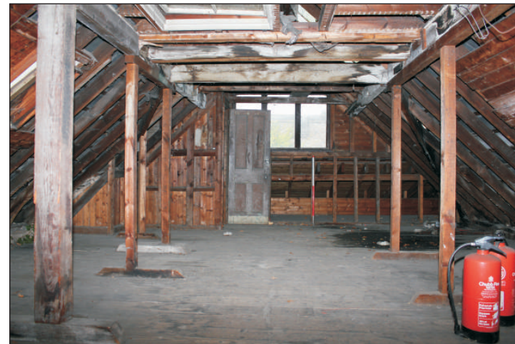
Plate 12: The first floor over room 5, viewed from the south. 1m scale.
