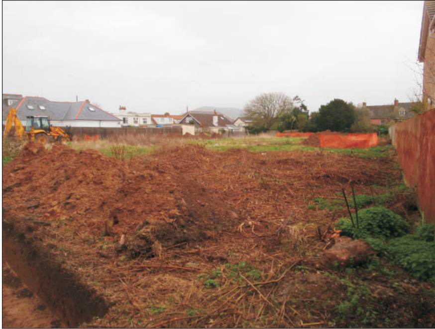
Plate 1: General view of site, looking northeast
