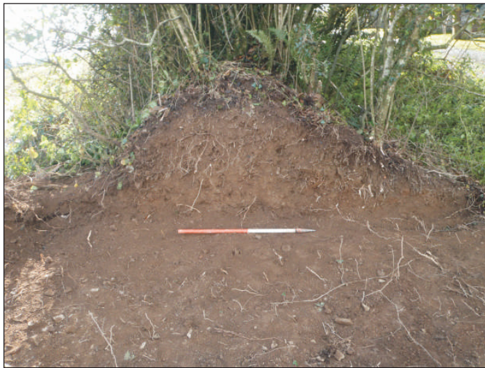
Plate 2: Hedgebank breach 2 viewed from the north. 1m scale.
