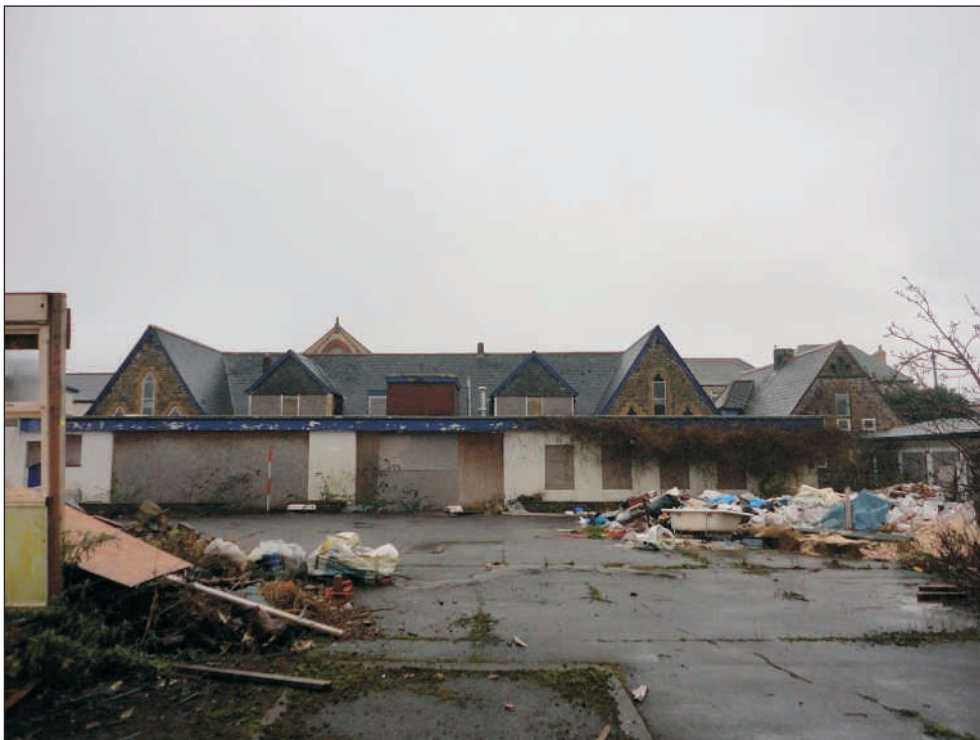
Plate 15: View from rear of school showing demolished prefabricated classrooms. 2m scale
