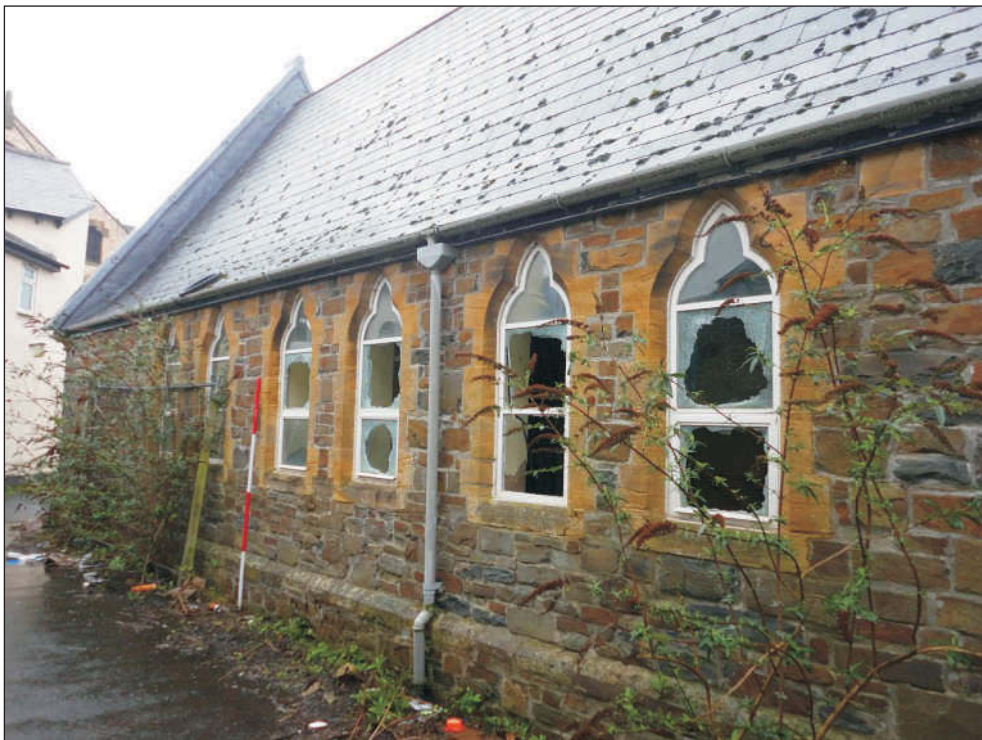
Plate 12: Short lancets on side walls, now blocked in northern and Infant's schoolroom. 2m scale
