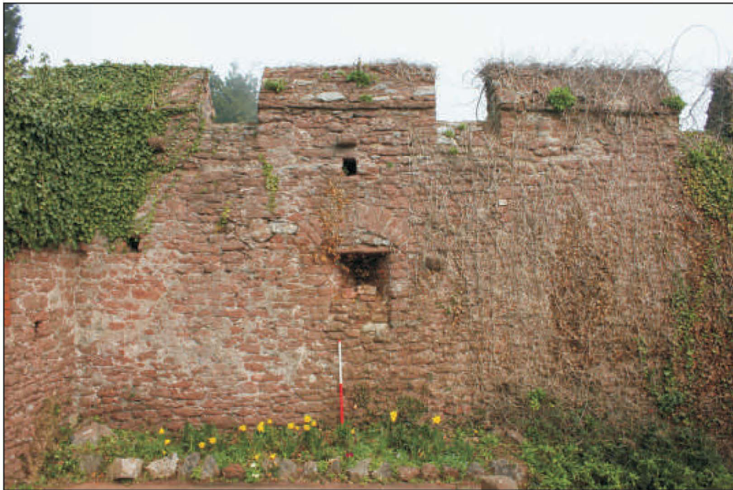
Plate 8: Wall F607, east internal elevation, viewed from the west. 1m scale.
