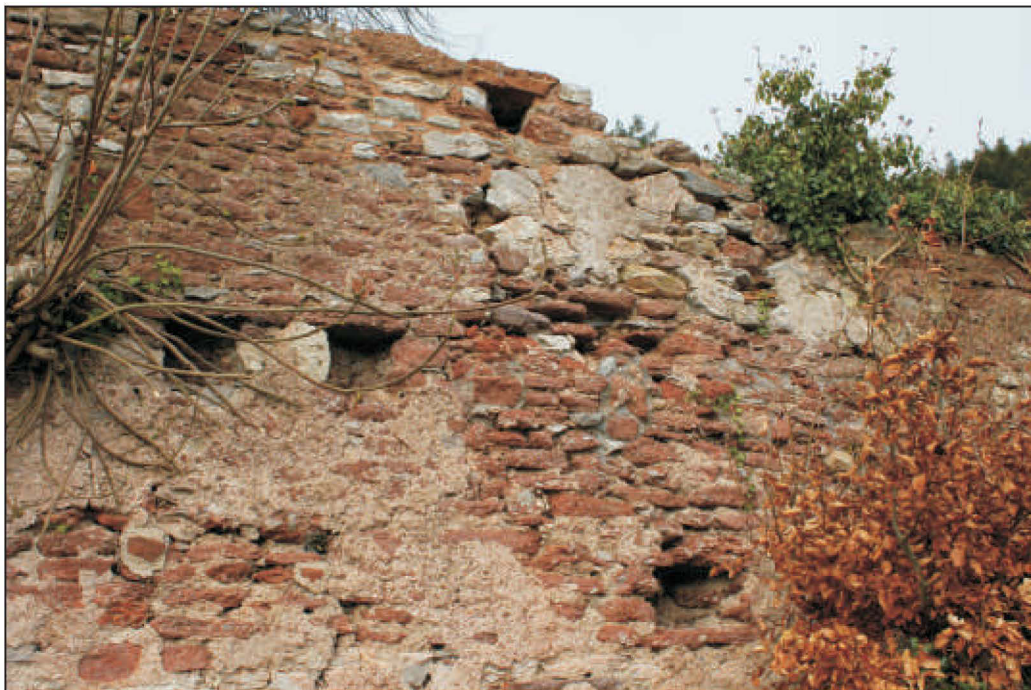
Plate 6: Joist sockets of first floor in F303, viewed from the southwest.
