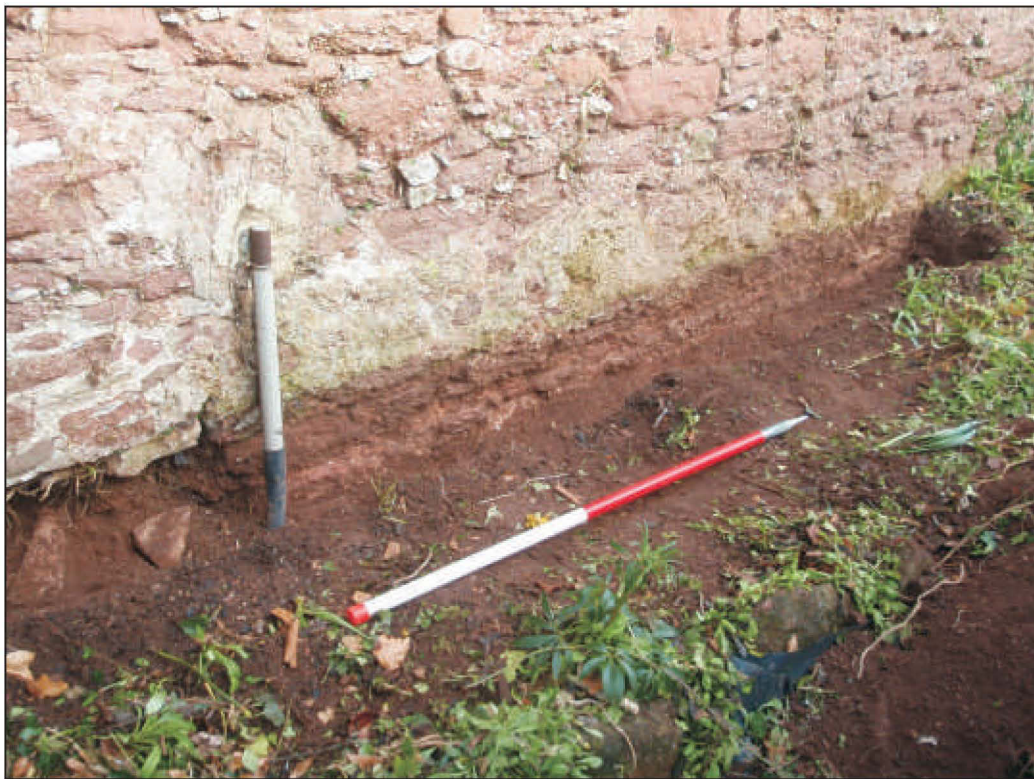
Plate 2: Flush footings of F303 to right, overlying rougher footings of F600, viewed from the southwest. 1m scale.
