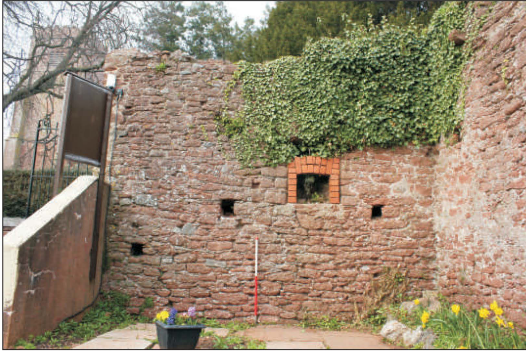
Plate 7: Wall F607, south internal elevation, viewed from the south. 1m scale.
