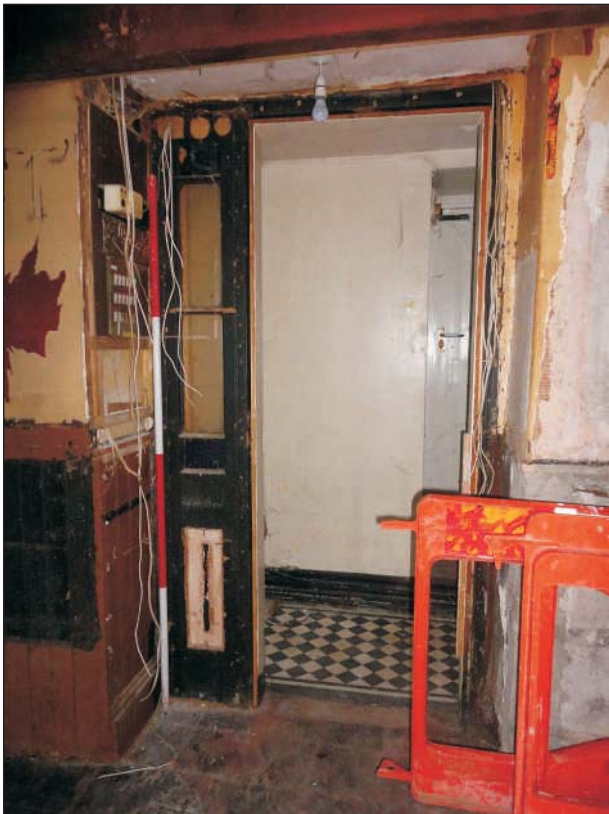
Plate 9: The remains of a glazed screen separating the corridor and staircase from the main bar. 2m scale
