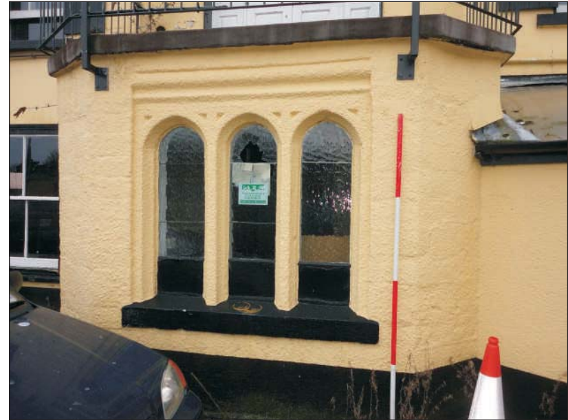
Plate 2: Detail of the reused late-medieval bay window built into the porch. 2m scale
