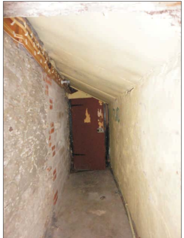
Plate 10: The curious, tunnel-like room in the rear lean-to, looking east
