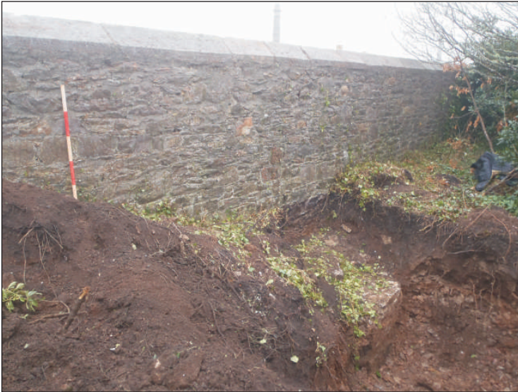
Plate 1: Test Pit 4 showing the yard boundary wall (2) and its projecting footings, viewed from the southwest. 1m scale.
