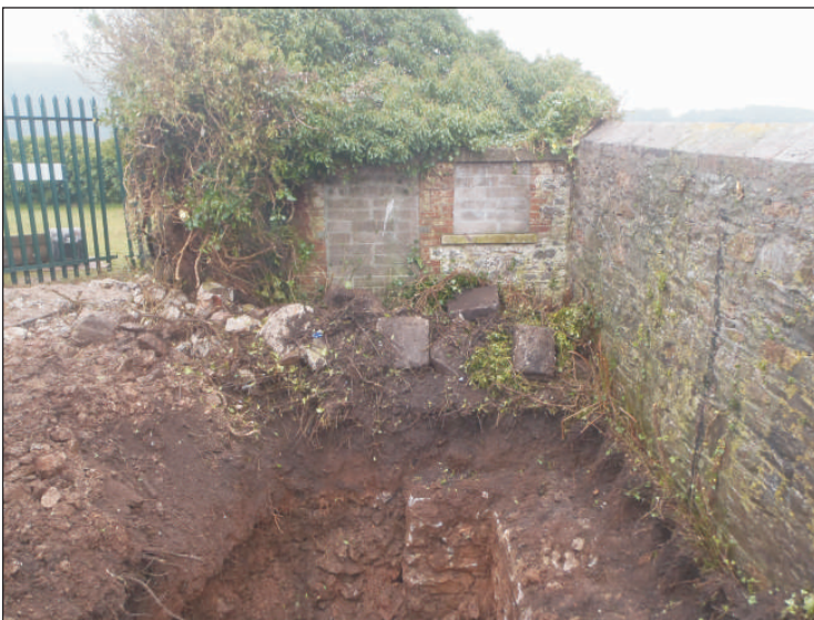
Plate 2: Test pit 4 showing the footings of the yard wall, with the northern part of upstanding wall 1 in the background, viewed from the east.
