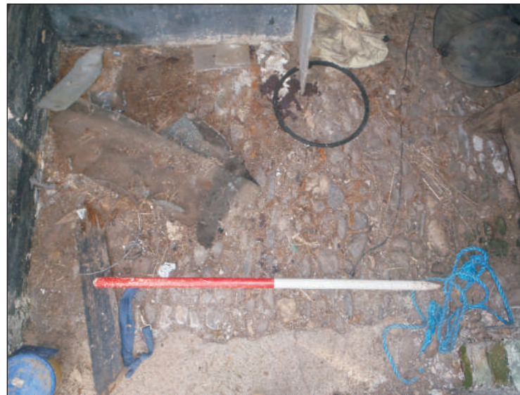
Plate 6: Pebble-lain floor surface of SSE ground floor room. View to ESE. Scale 1m
