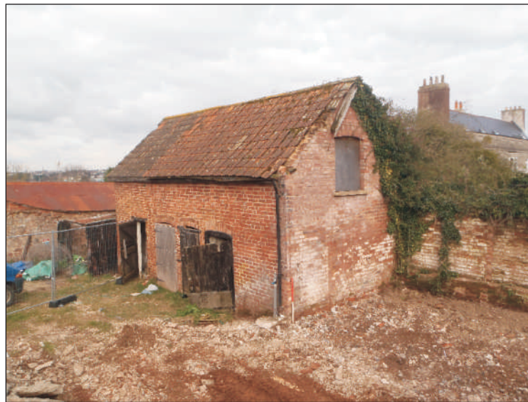
Plate 3: View of brick structure, looking south. Scale 1m
