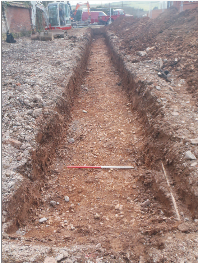
Plate 1: Trench 1, general view, looking SSW. Scale 1m
