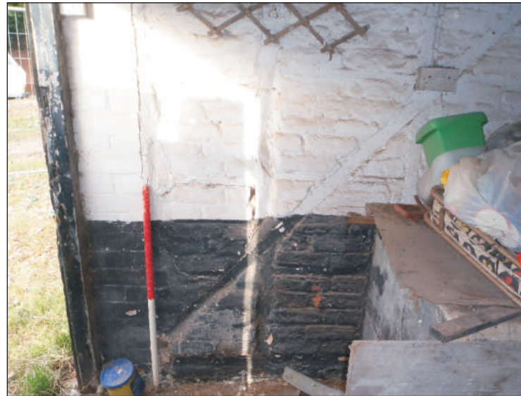
Plate 5: Timber frame and brick nogging partition, looking NNE. Scale 1m
