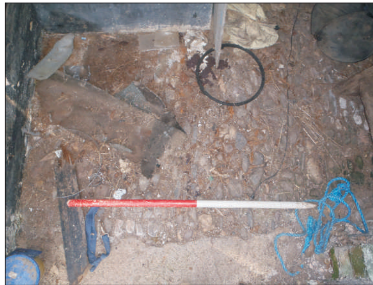
Plate 6: Pebble-lain floor surface of SSE ground floor room. View to ESE. Scale 1m
