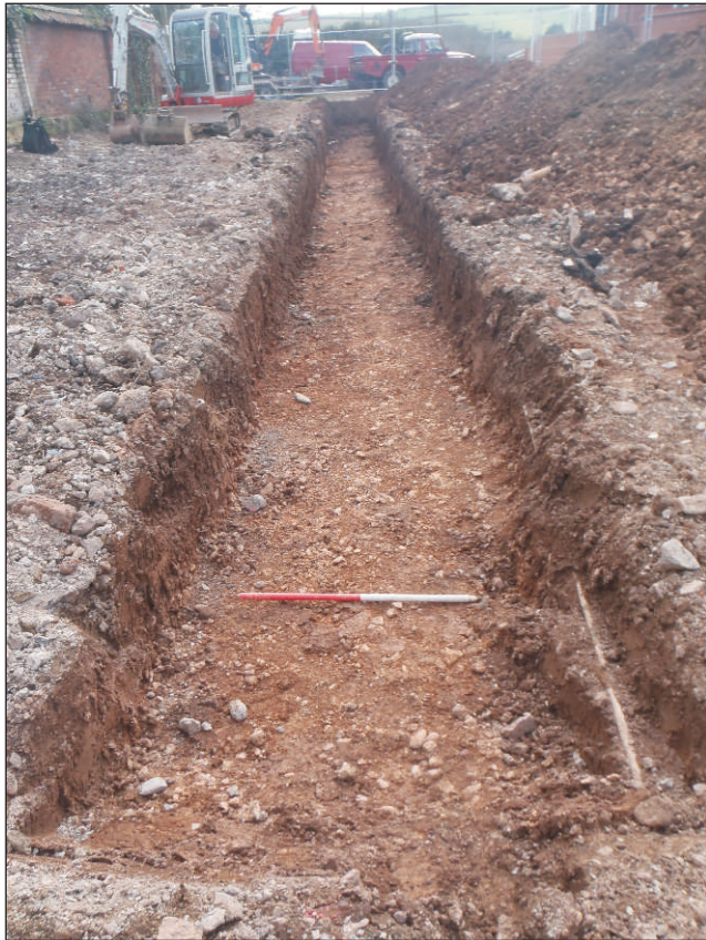
Plate 1: Trench 1, general view, looking SSW. Scale 1m
