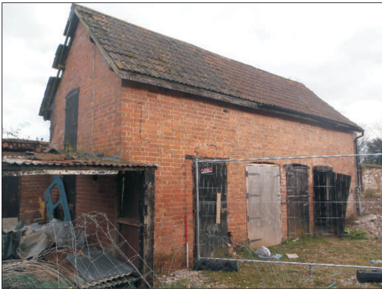
Plate 4: View of brick structure, looking south. Scale 1m
