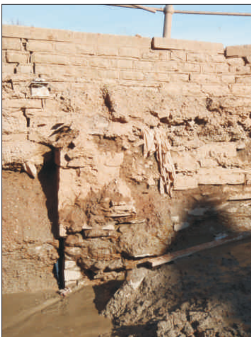
Plate 6: Wall 7 viewed from the west.
