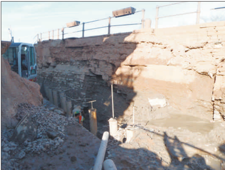
Plate 5: Wall 6 viewed from the southwest.
