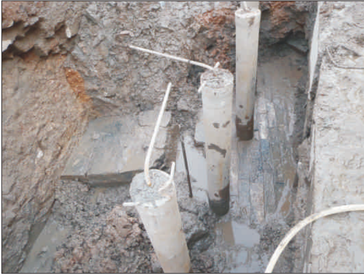
Plate 4: Surface 2, viewed from the north.
