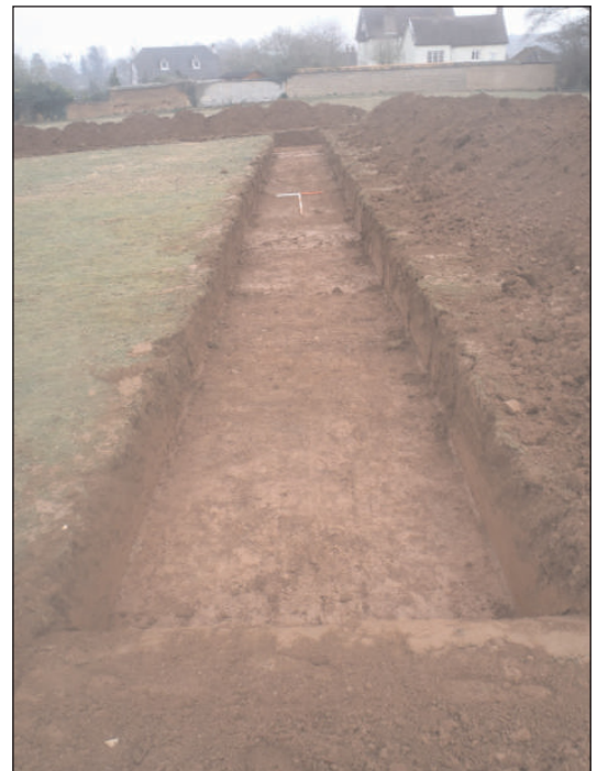
Plate 8: General view of Trench 14, view from west (scale 2m x 1m)
