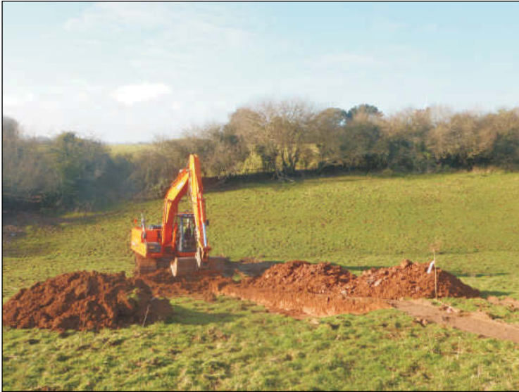
Plate 1: General view of Area 1, with Area 2 beyond the hedgeline
