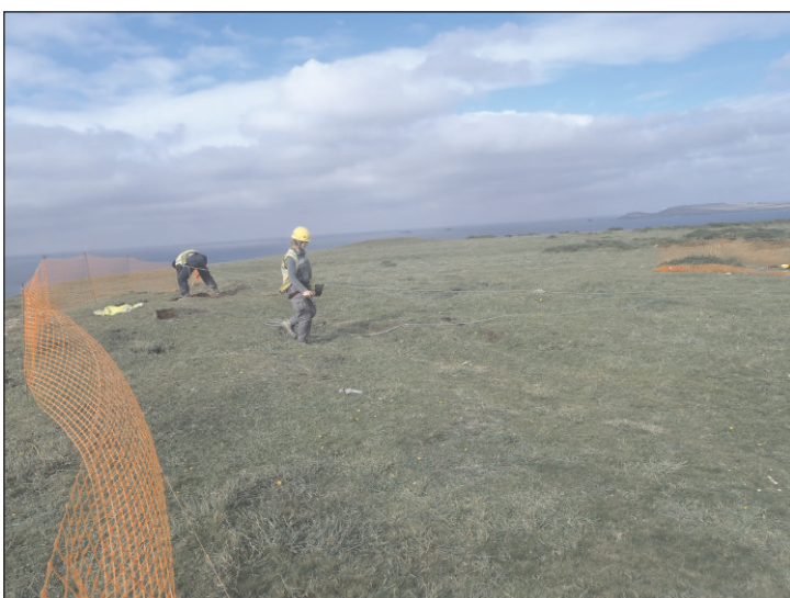
Plate 3: Working shot of de-turfing, view from the SE
